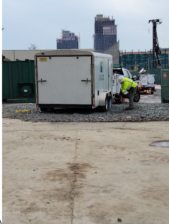
Photo 1- Reresnattive photo of Cascade demobilizing equipment. .
