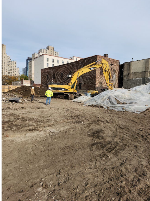
Photo 1- Representative photo of excavation work in the northern portion of the Site (formerly Lot 15).
