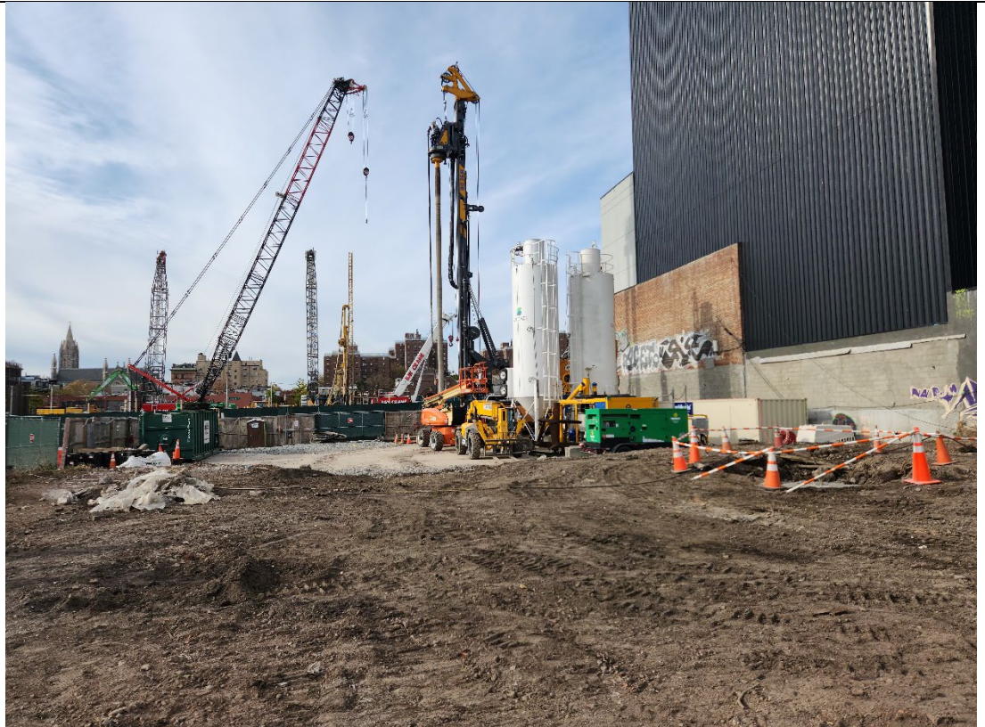
Photo 2 – Representative photo of of the Site facing northwest towards Nevins Street.
