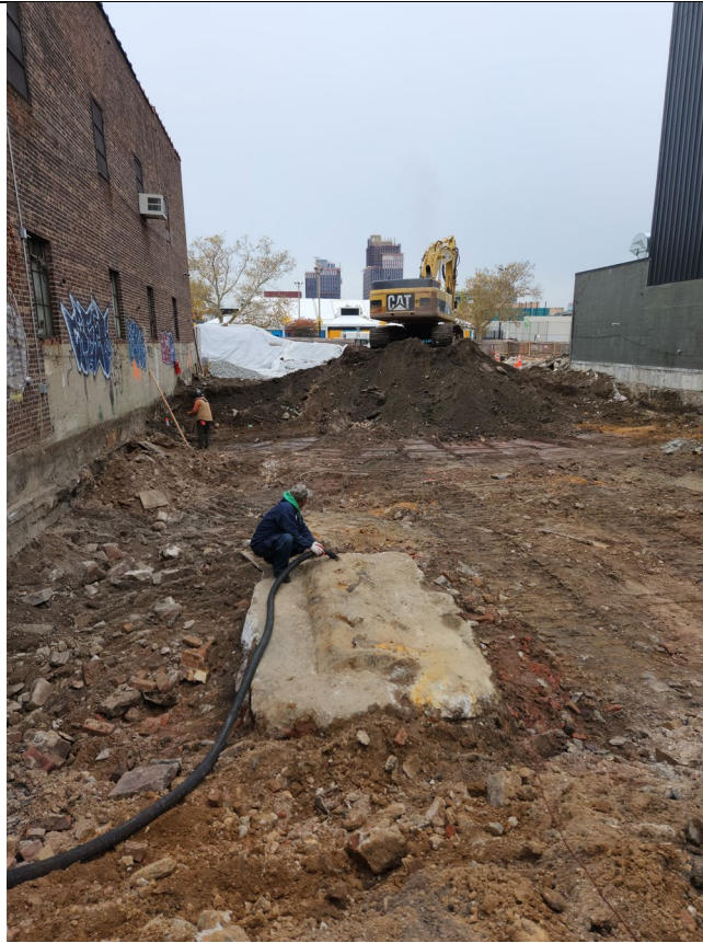
Photo 3- Photo of ABC Tank pumping liquid from concrete encased UST located in grids A7 and B7.
