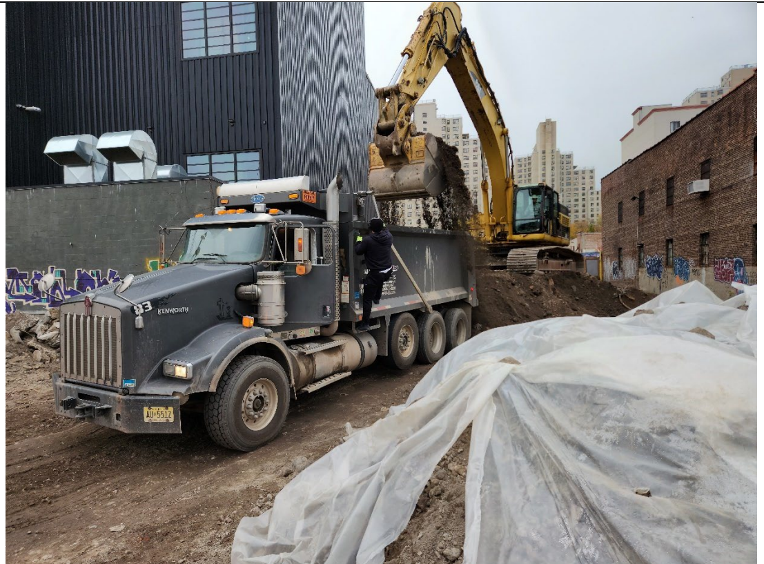
Photo 2 – Representative view of material load out for off-Site disposal to Bayshore.
