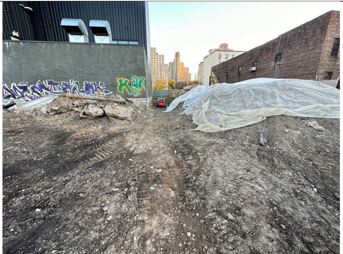
Photo 2 – Representative view of the Site facing northeast from Douglass Street.
