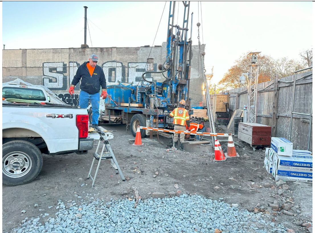
Photo 4 – Representative view of the east side of Site during drillign activities.
