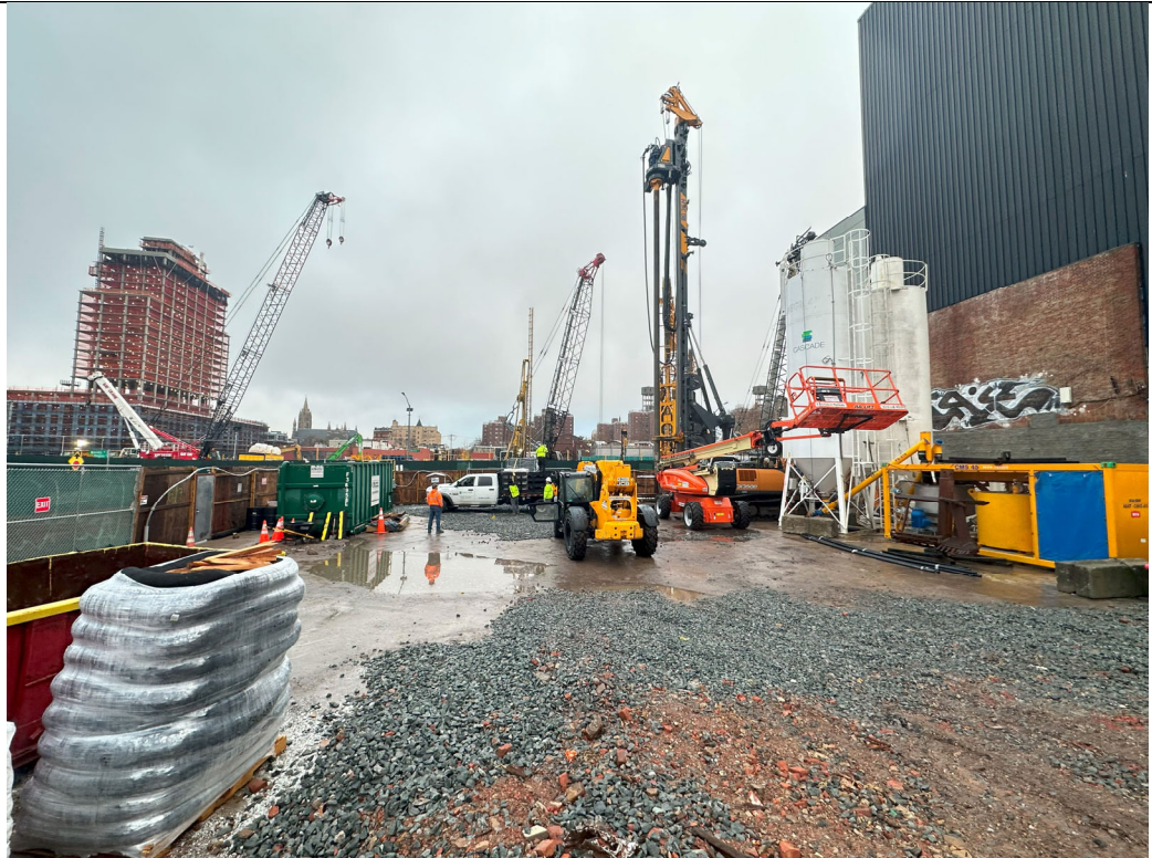
Photo 2 – West side of site, Cascade unloading pallet of cement.
