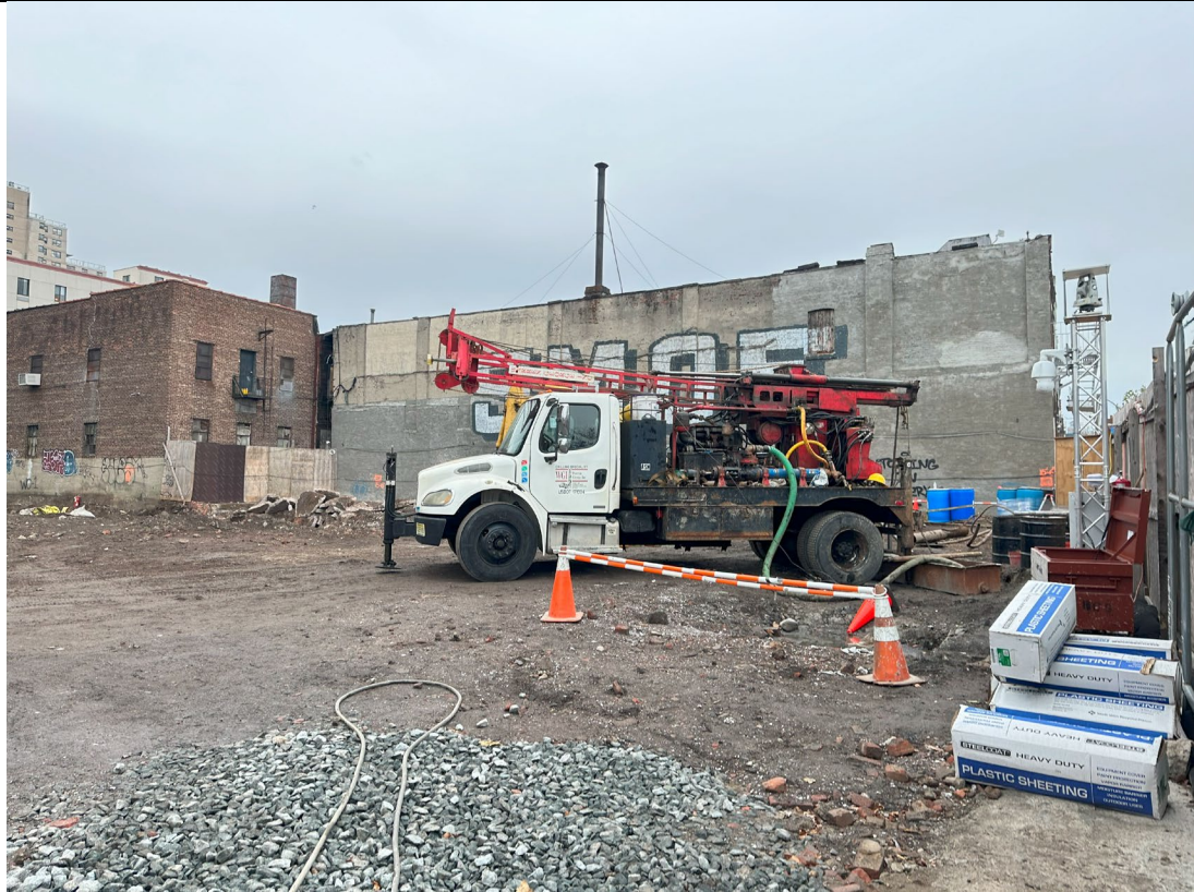
Photo 5- Representative view of GES mobilized at Mix C (Columns 23, 24, and 25).
