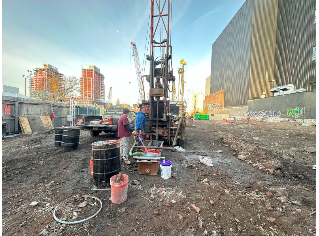
Photo 1- Representative photo of GES beginning mud rotary/split spoon sampling within overlap boring for Mix A, Columns: 154, 155 and 102.
