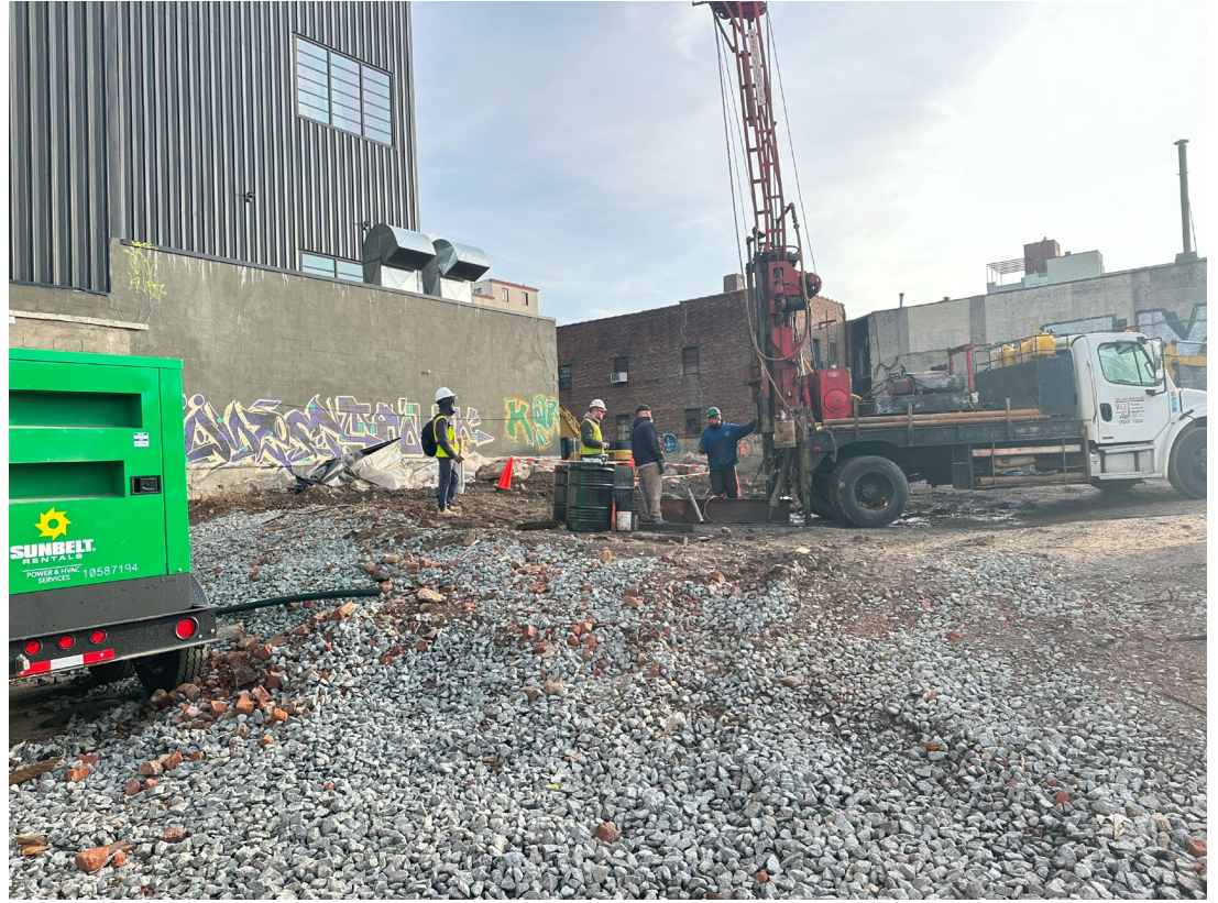
Photo 1- Representative view of ISS-B-1 being advanced at overlap of Columns 304 and 337 (Mix B).
