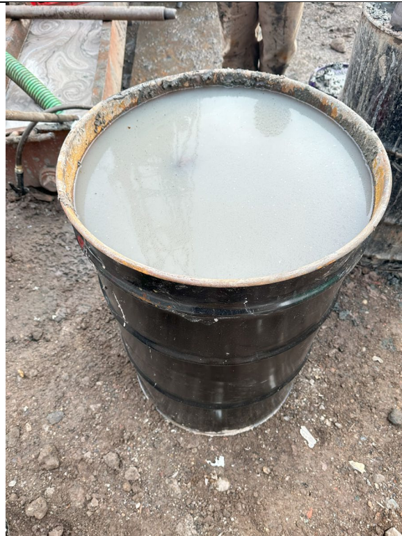
Photo 2 – Representative view of liquid from rid mud pan being drummed following the completion boring for Mix B.
