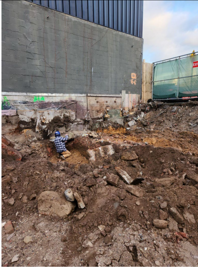
Photo 5- Additional view of old brick foundation in WC- 1.
