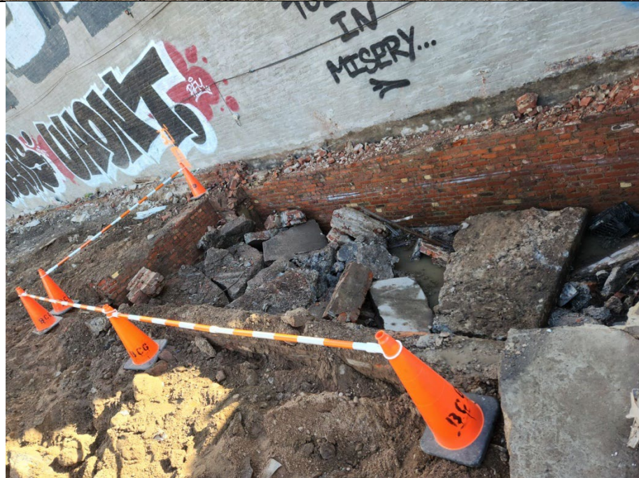
Photo 2 – .Representative photo of former partial cellar located on the eastern portion of the property.
