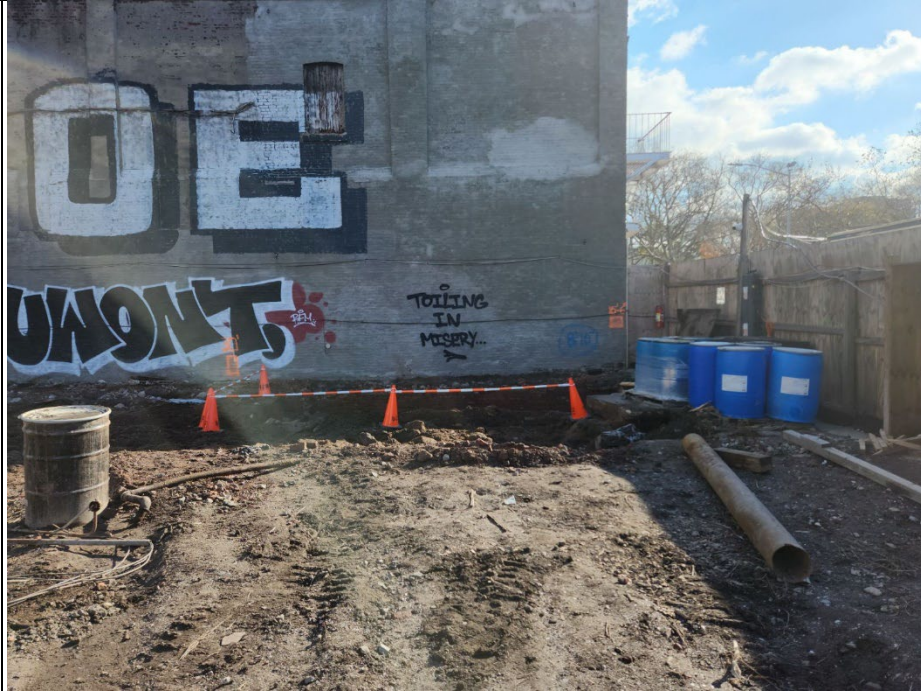
Photo 1- Representative photo of eastern portion of the Site.
