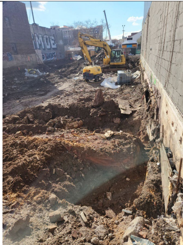
Photo 4 – Representative photo of old brick foundation in WC- 1.
