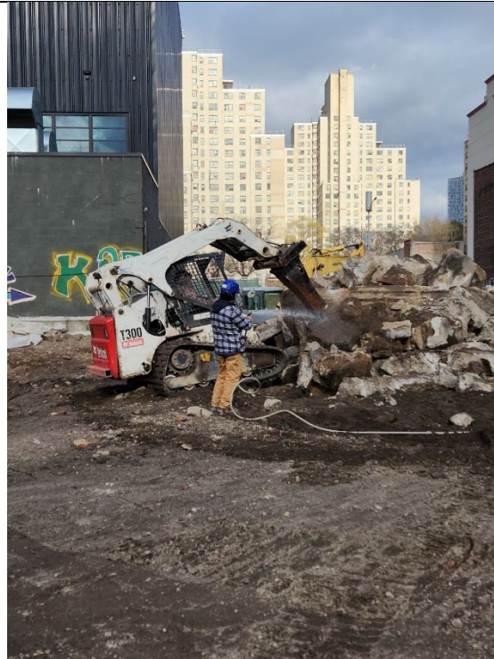
Photo 3- Representative photo of concrete being broken down into smaller pieces.
