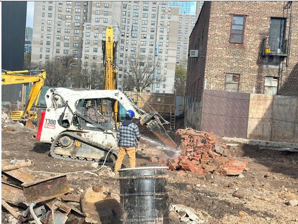
Photo 5- Representative photo of brick being broken up and active dust suppression.
