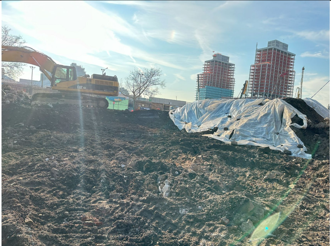
Photo 4- Representative view of excavated material from WC- 4, covered with poly at the end of the day.
