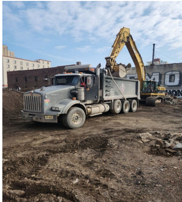
Photo 2 – Representative view of truck being loaded wit concrete for disposal at PPark.
