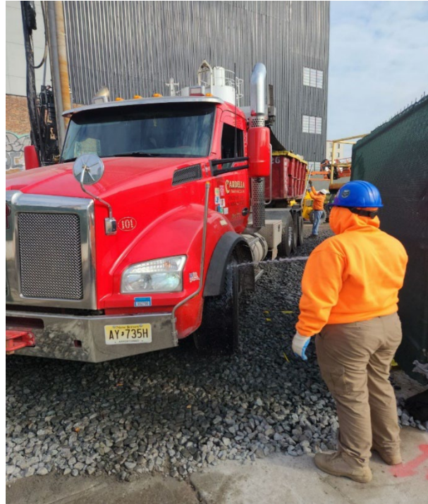
Photo 1- Representative view of tires wash over track pad.
