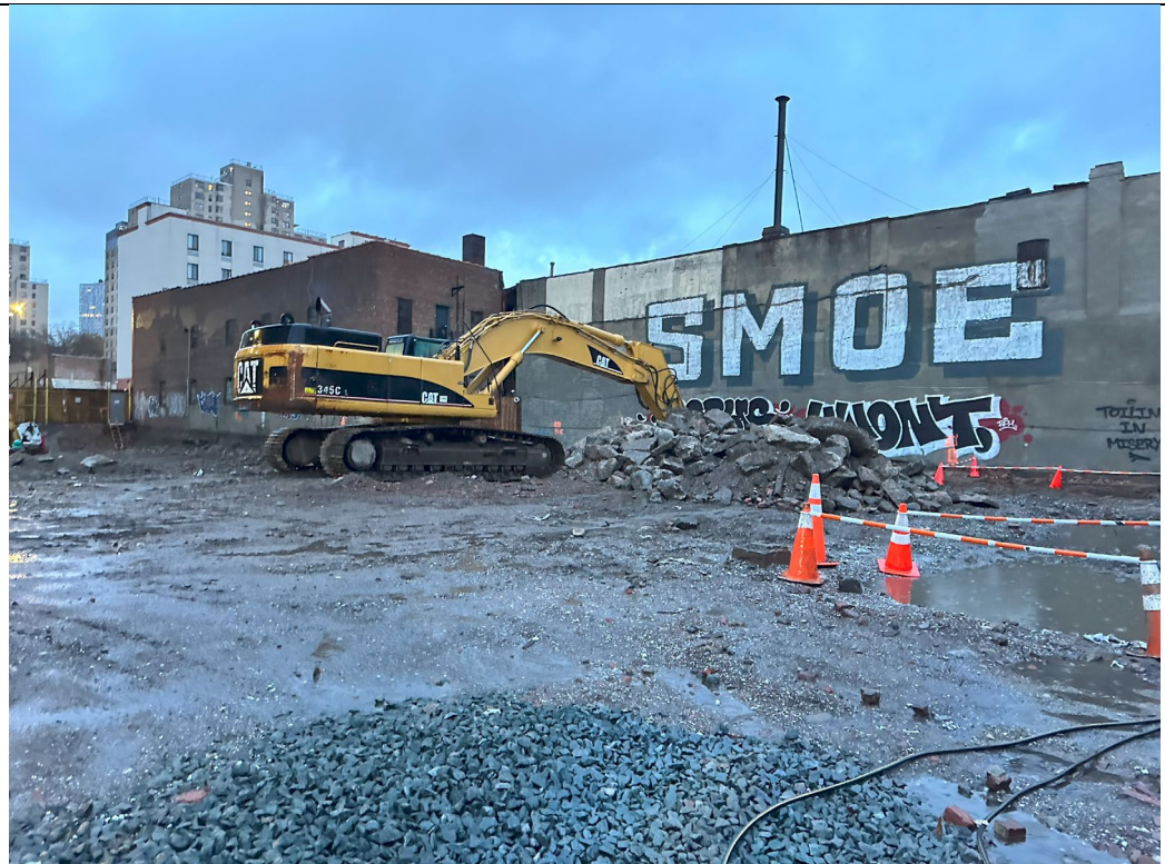
Photo 2 – Representative view excavating WC4 to load on trucks.
