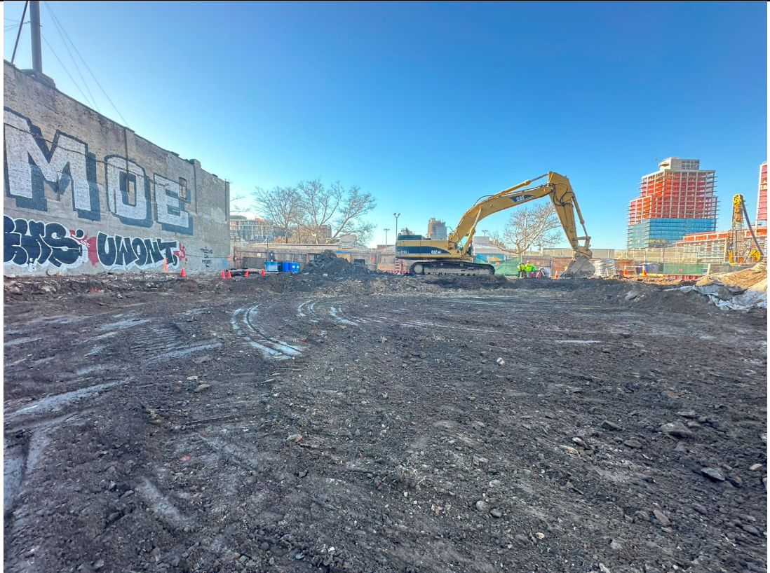
Photo 3- Representative view of southeast side of site.
