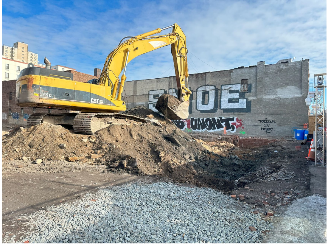
Photo 3- Representative view of excavation work within WC-7.
