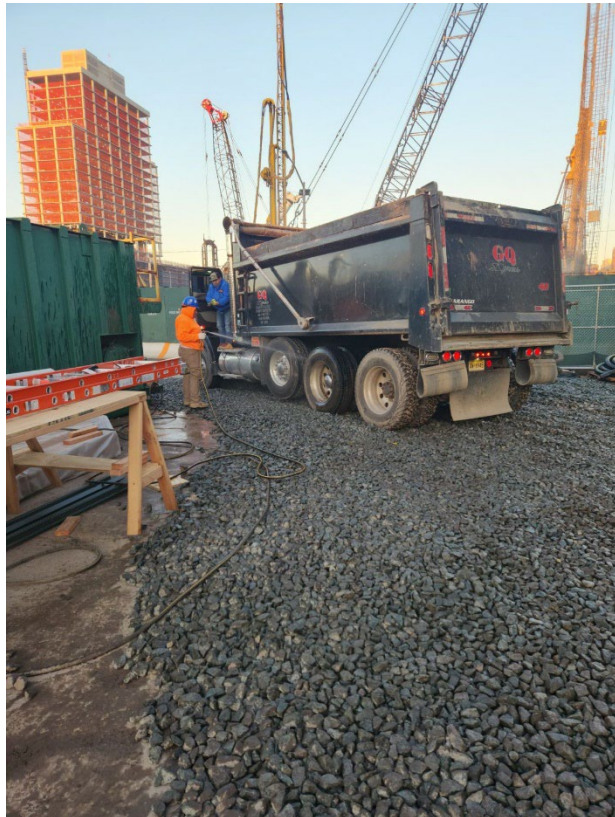
Photo 2 –Representative view of trucks tires being washed on truck wash pad.
