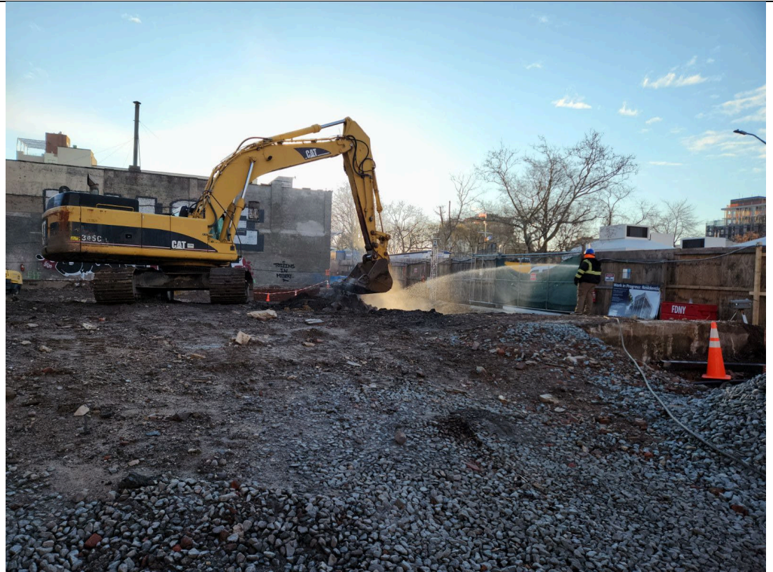
Photo 3- Representative view of excavation activities in WC-7 and active dust suppression.
