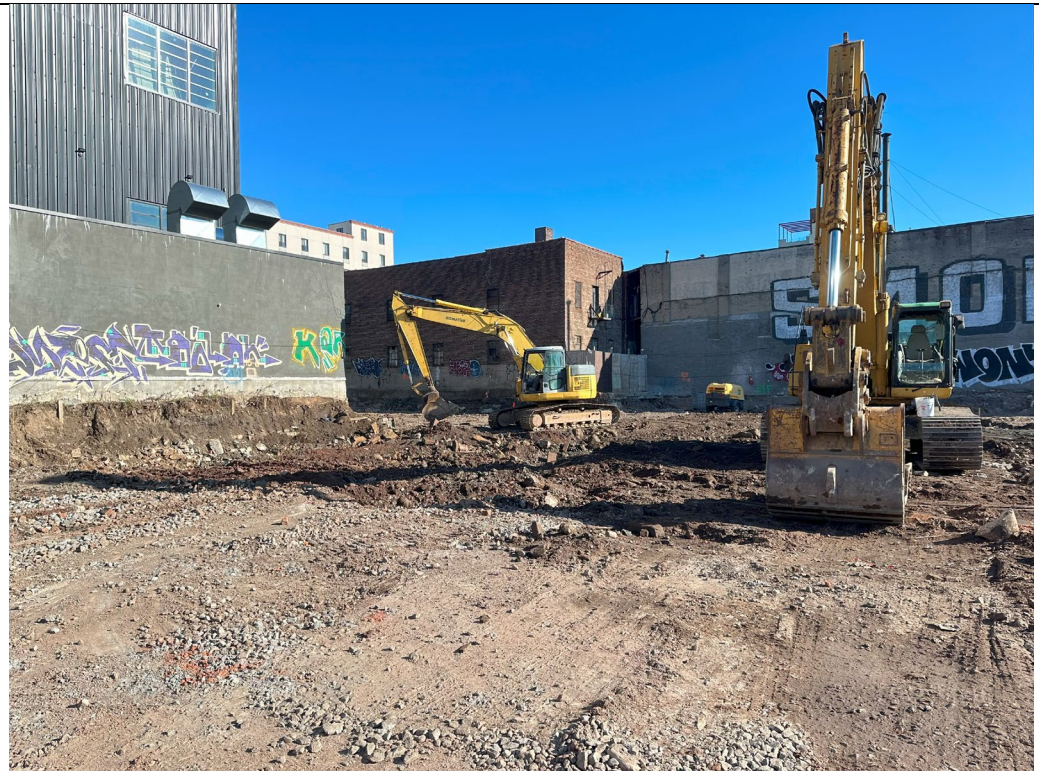
Photo 4- Representative view of excavator grading in WC-3.
