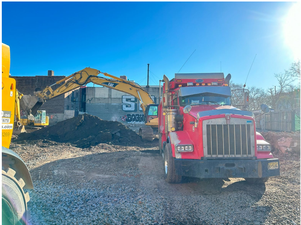
Photo 2 – Representative view of truck loading material for off-site disposal from WC-3.
