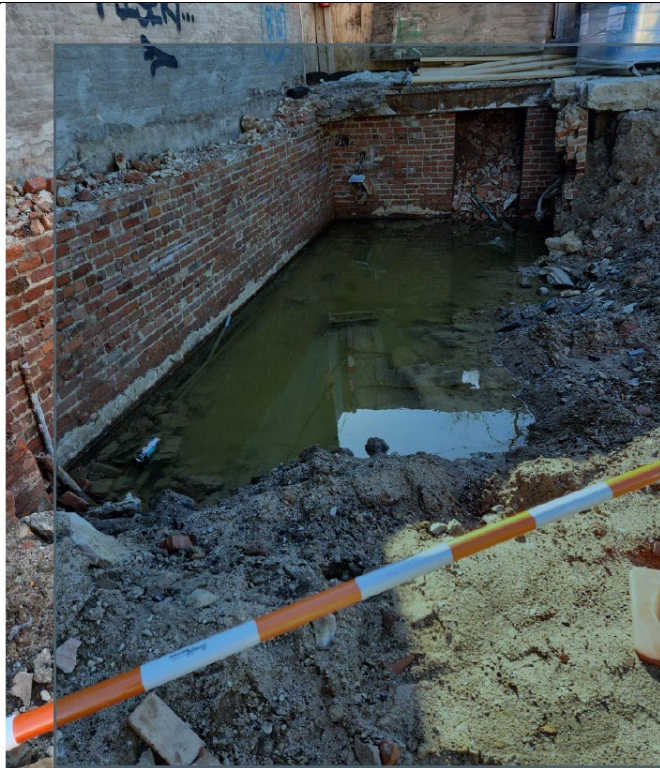
Photo 6- Representative photo of standing water in former building cellar.
