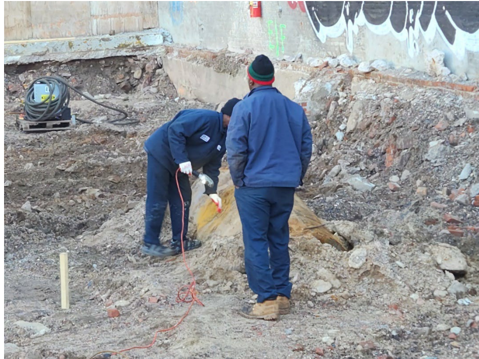
Photo 1- Representative photo of tank being cut open by ABC tank in order to pump out contents.
