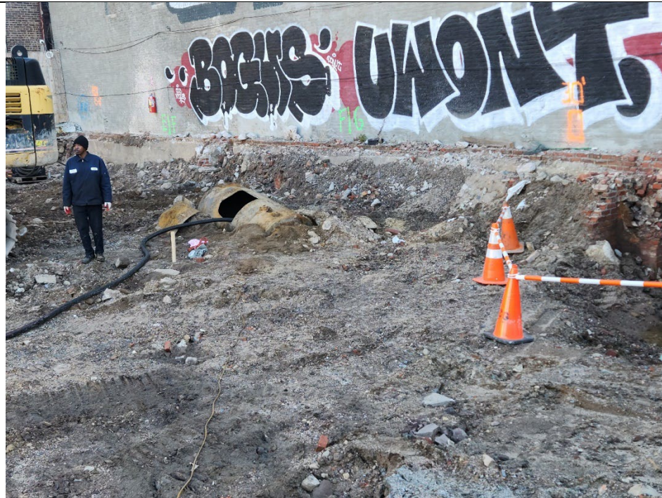
Photo 2 – Representative photo ABC Tank pumping out contents of UST.
