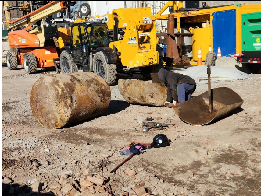
Photo 3- Representative photo of tank being cut and prepped for scrapping by ABC Tank.
