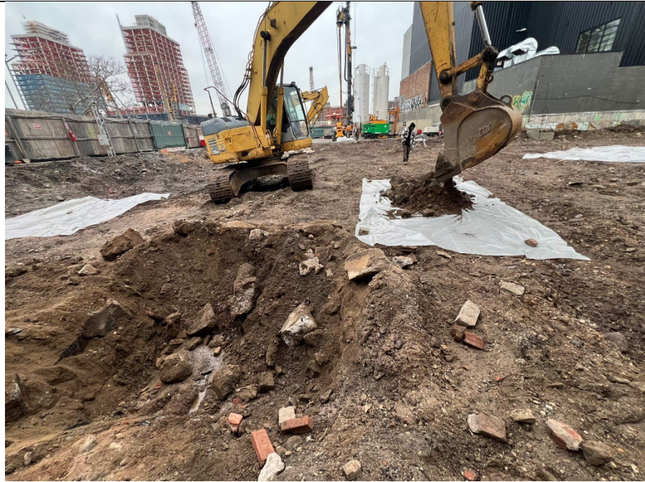
Photo 3 - Representative photo of excavated material being put on poly.
