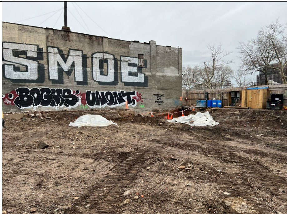
Photo 4 - Representative photo of stockpiled material covered with poly at the end of the day.
