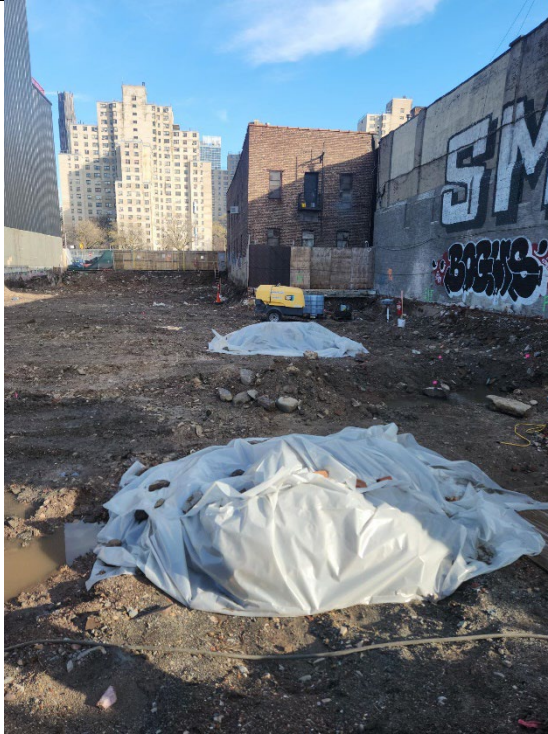
Photo 1 – Representative view of tank #2 area (furthest from camera) and arsenic hotspot, stockpiled soil (closest to camera).
