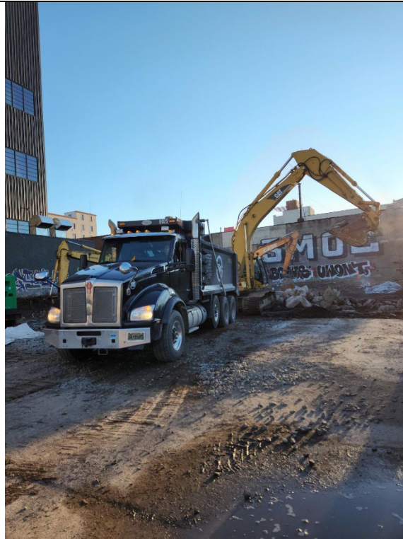
Photo 1 – Truck load out of concrete to Ppark.
