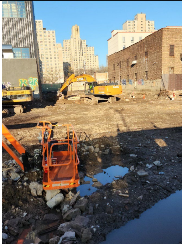
Photo 3 – Representative view of grading soil in northern area of the Site.
