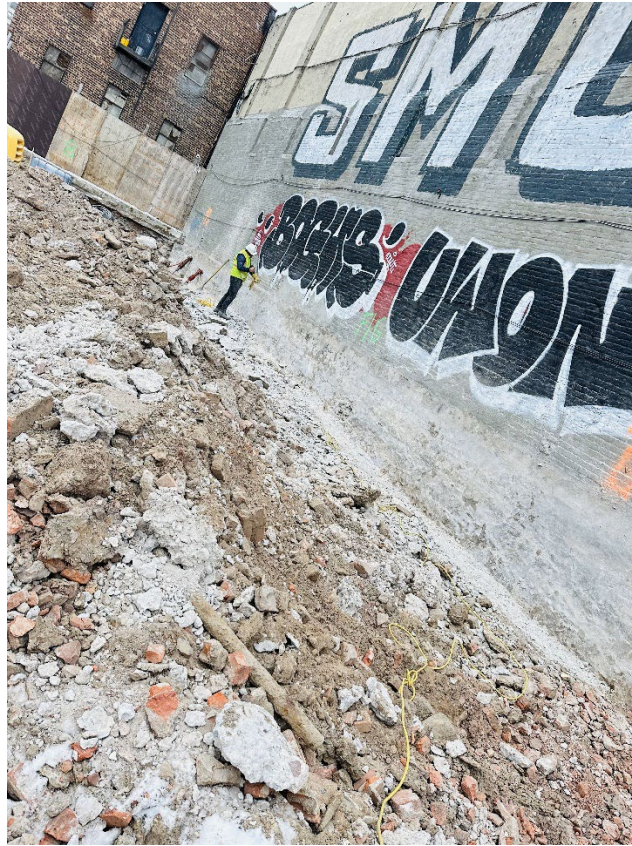
Photo 1 – Representative view of Xolle crew working on the eastern wall.
