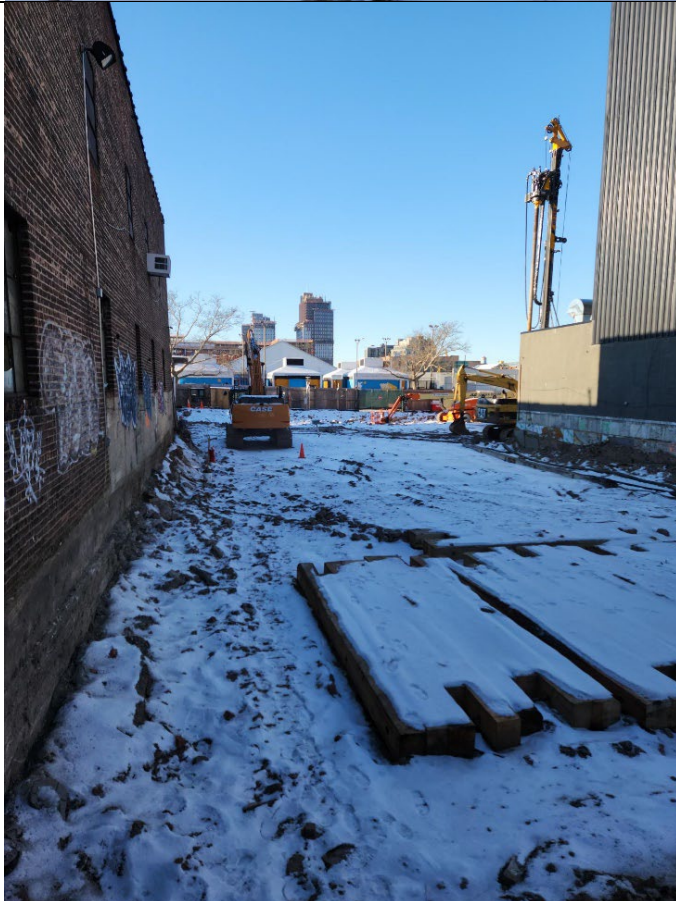
Photo 4 – Representative view of the Site facing south.
