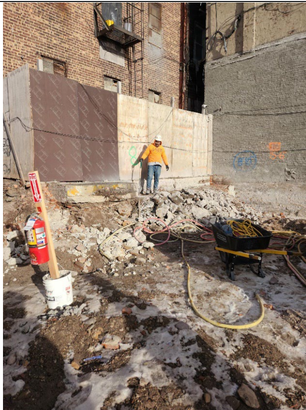
Photo 2 – Additional view of Xolle laborer jack hammering of ledge .
