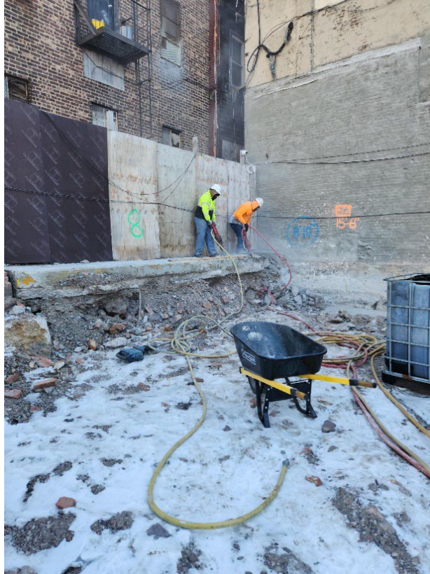
Photo 1 – Representative view of Xolle jack hammering ledge.
