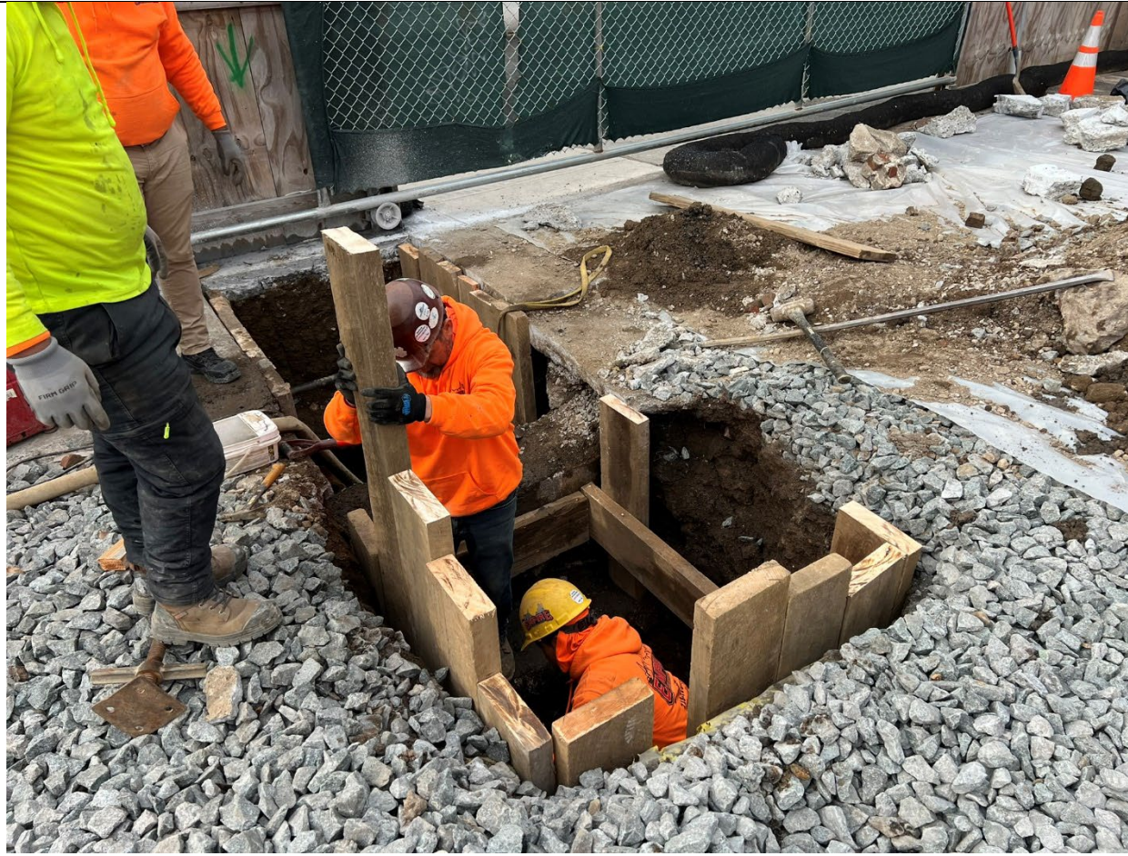
Photo 3- Representative view of work on the sewer connection.
