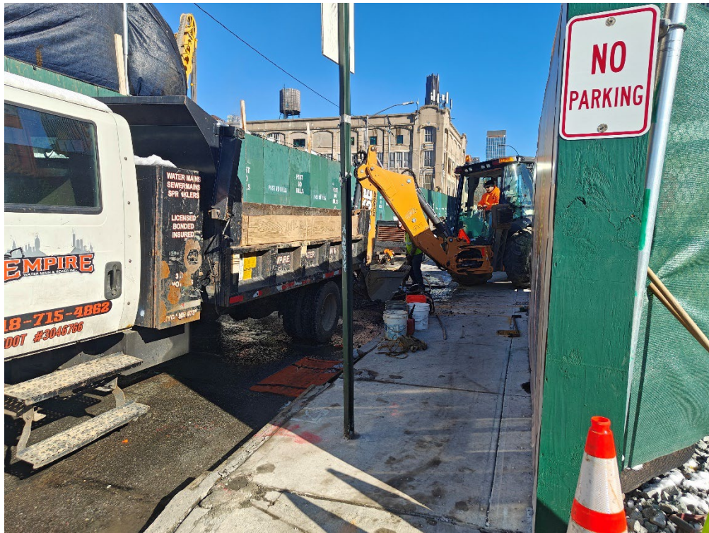
Photo 2 – Representative view of plumbers working on Nevins Street.
