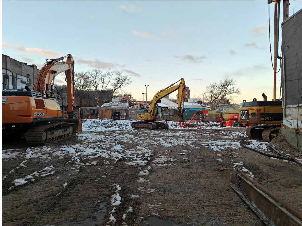
Photo 1- Representative view of the Site facing south.
