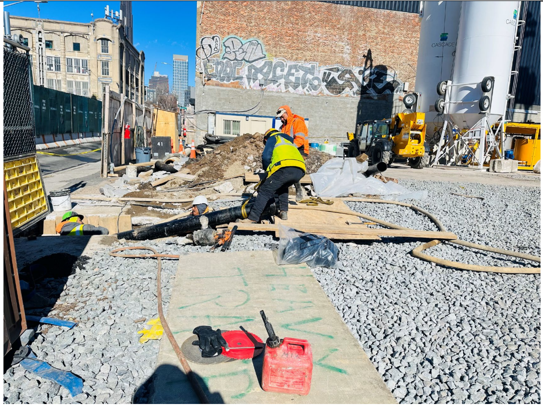
Photo 3- Representative view of pipe being installed.
