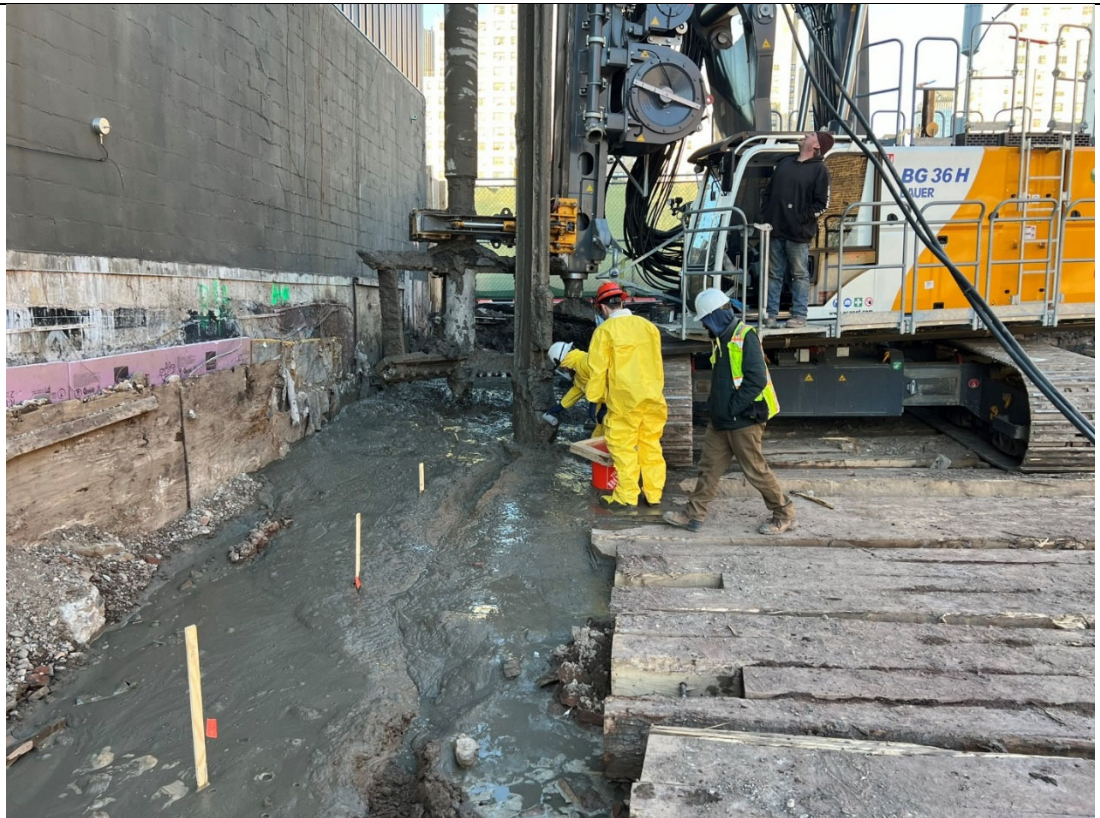
Photo 4- Representative photo of grabbing a wet mix sample from ISS column 650.
