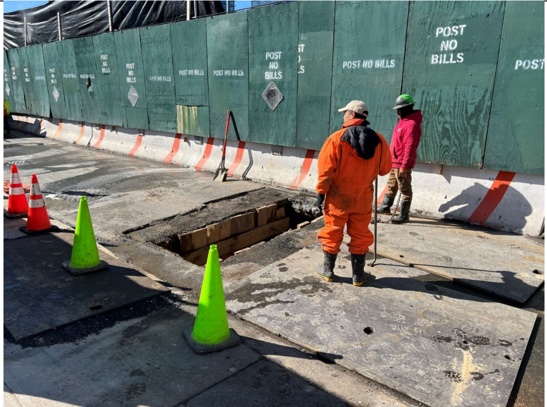
Photo 5- Representative photo of the sewer connection work on Nevins Street.
