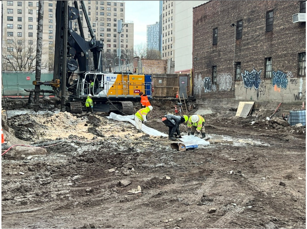
Photo 5- Representative photo of poly being laid for the decontamination of the sampling tool.
