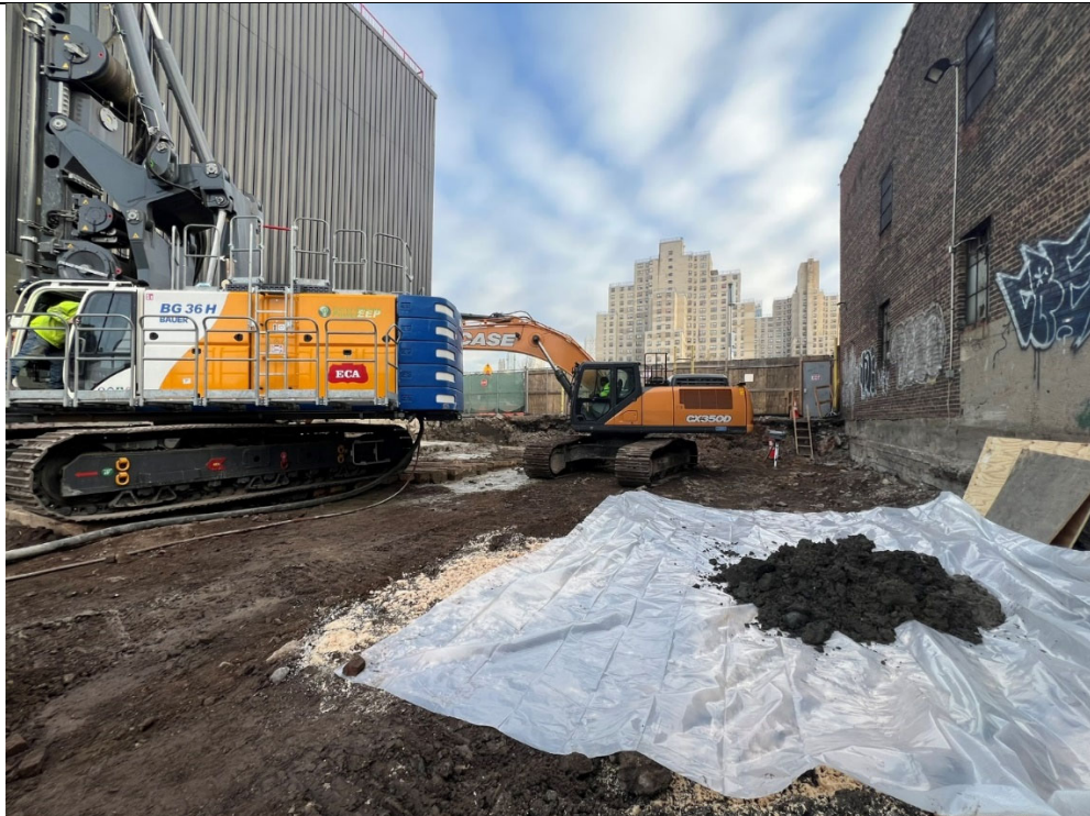
Photo 2 – Representative photo of swell material being stockpiled on poly.
