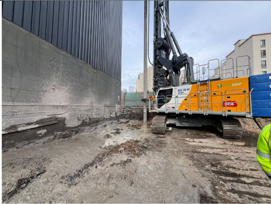
Photo 3- Representative photo of drilling an ISS column.
