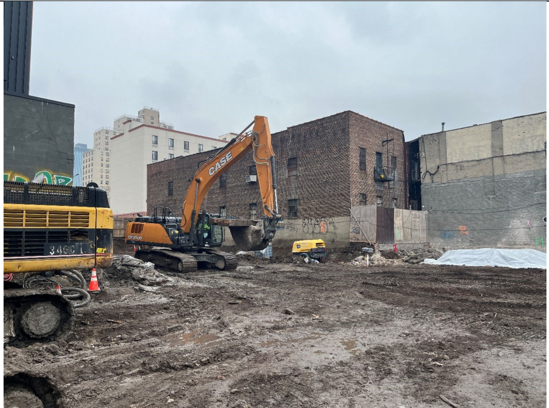
Photo 3- Representative photo of Cascade moving equipment from northern portion of the site.
