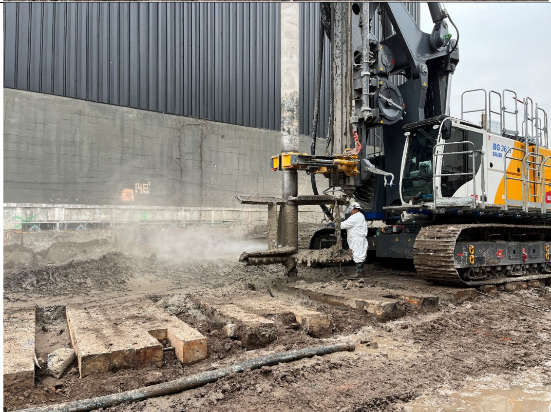
Photo 2 – Representative photo of auger cleaning after drilling activities were halted.
