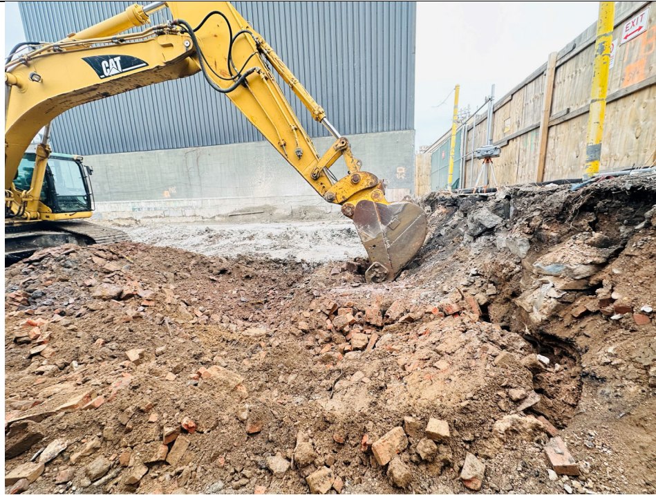
Photo 1- Representative photo of excavator working on removal of obstructions.
