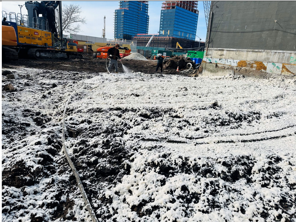
Photo 4- Representative photo of WC-1 work zone sprayed with ATMOS foam.
