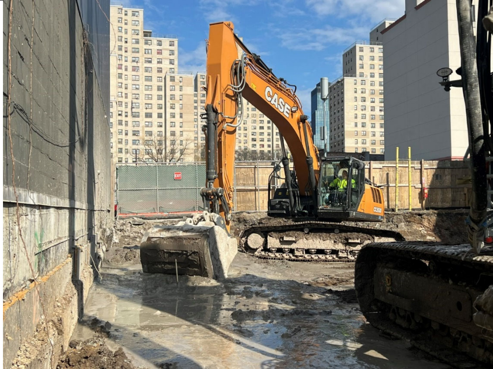
Photo 1- Representative photo of attempting to remove obstructions from columns 581 and 598.
