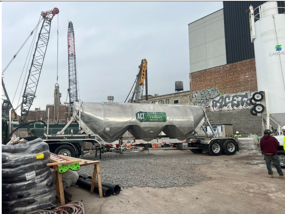
Photo 4- Representative photo of slag being delivered to the Site for the batch plant.
