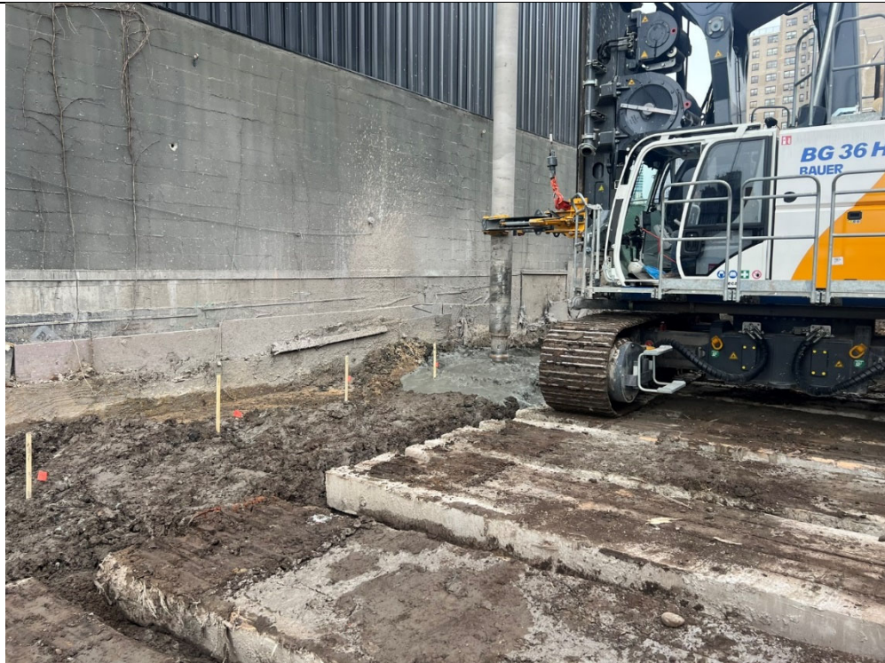
Photo 2 – Representative photo of installing an ISS column.
