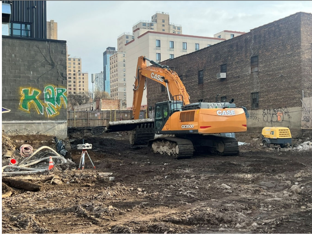
Photo 5- Representative photo of the stabilizing mats being moved to the northern portion of the Site.
