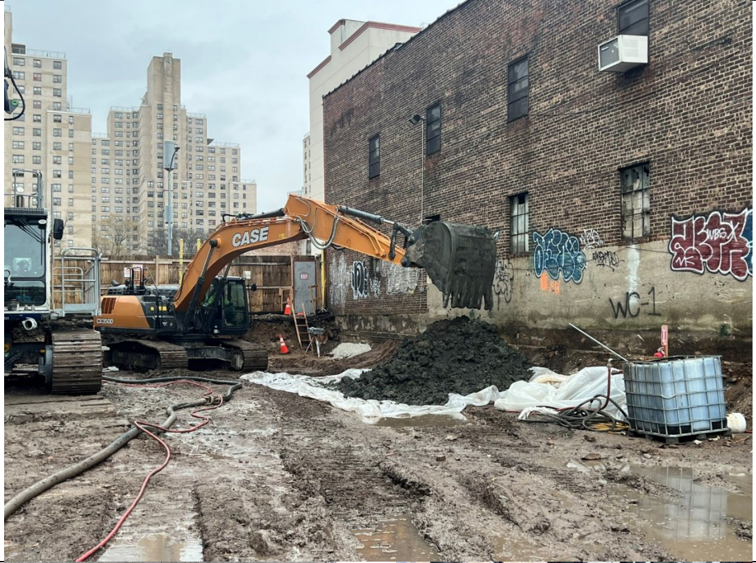
Photo 1- Representative photo of Cascade stockpiling the swell material on poly, this material will be tested prior to disposal.
