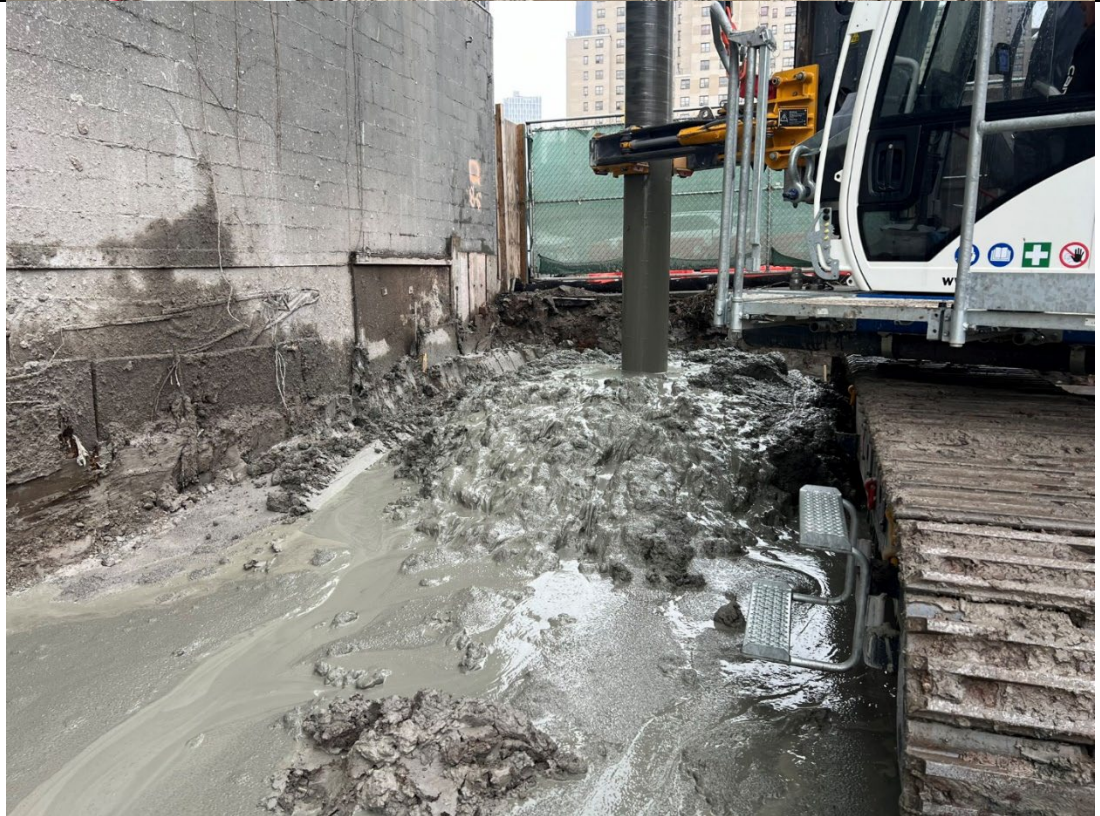
Photo 2 – Representative photo of ISS column installation.
