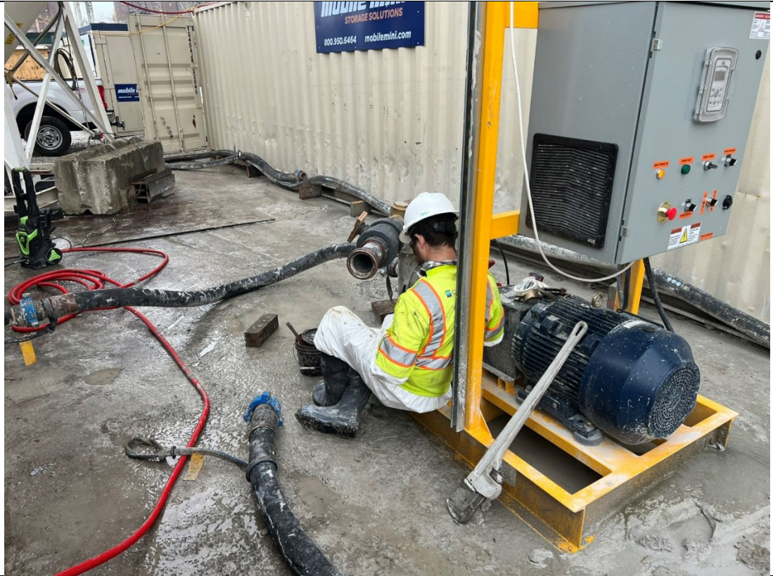
Photo 3- Representative photo of Cascade working on pump.
