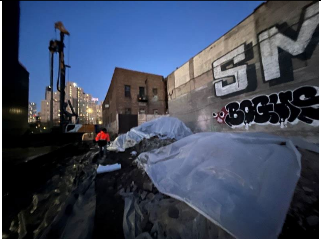
Photo 5- Representative photo of stockpiled material covered at the end of the workday.
