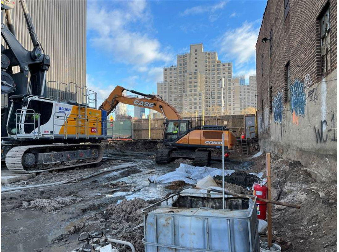
Photo 1- Representative photo of Cascade stockpiling the swell material on poly, this material will be tested prior to disposal.
