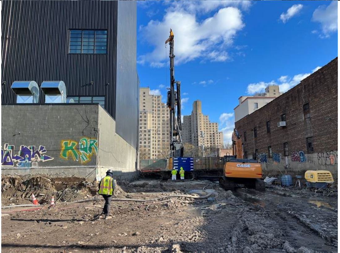
Photo 2 – Representative photo of ISS column installation.
