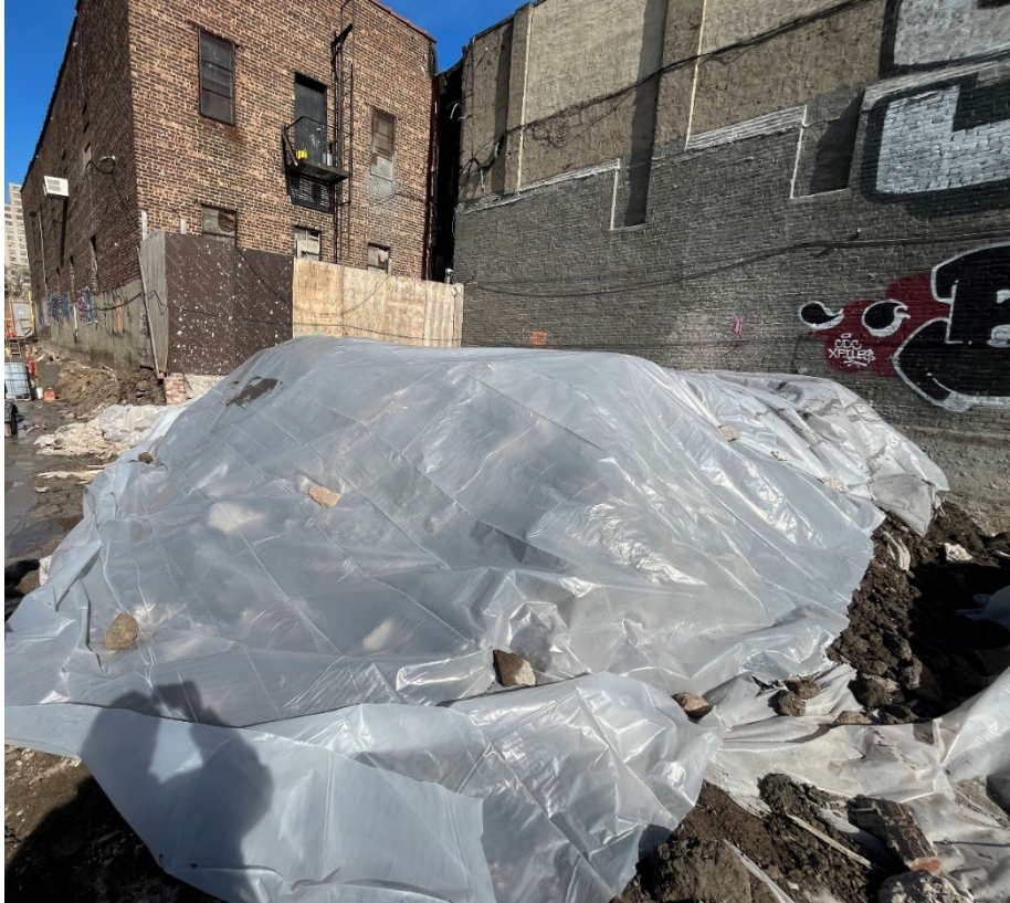
Photo 4- Representative photo of stockpiled material covered at the end of the workday.
