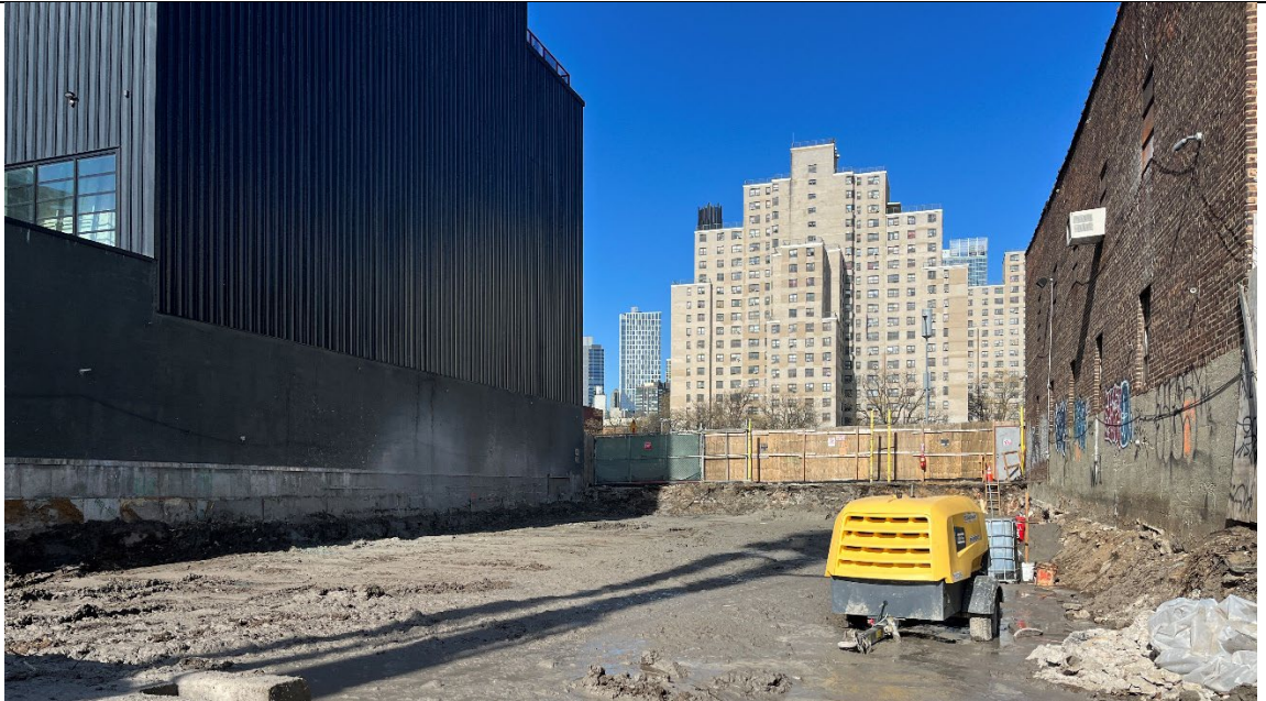
Photo 3- Representative photo of northern lot at the end of the workday.
