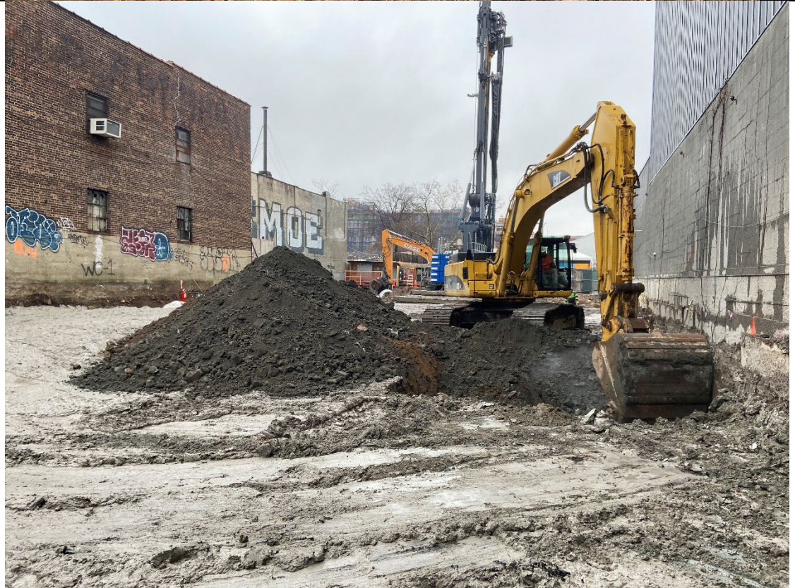
Photo 2 – Representative photo of excavation to expose obstruction.
