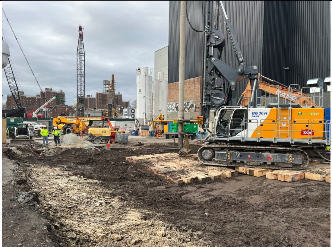
Photo 5- Representative photo of the site at the end of the day.
