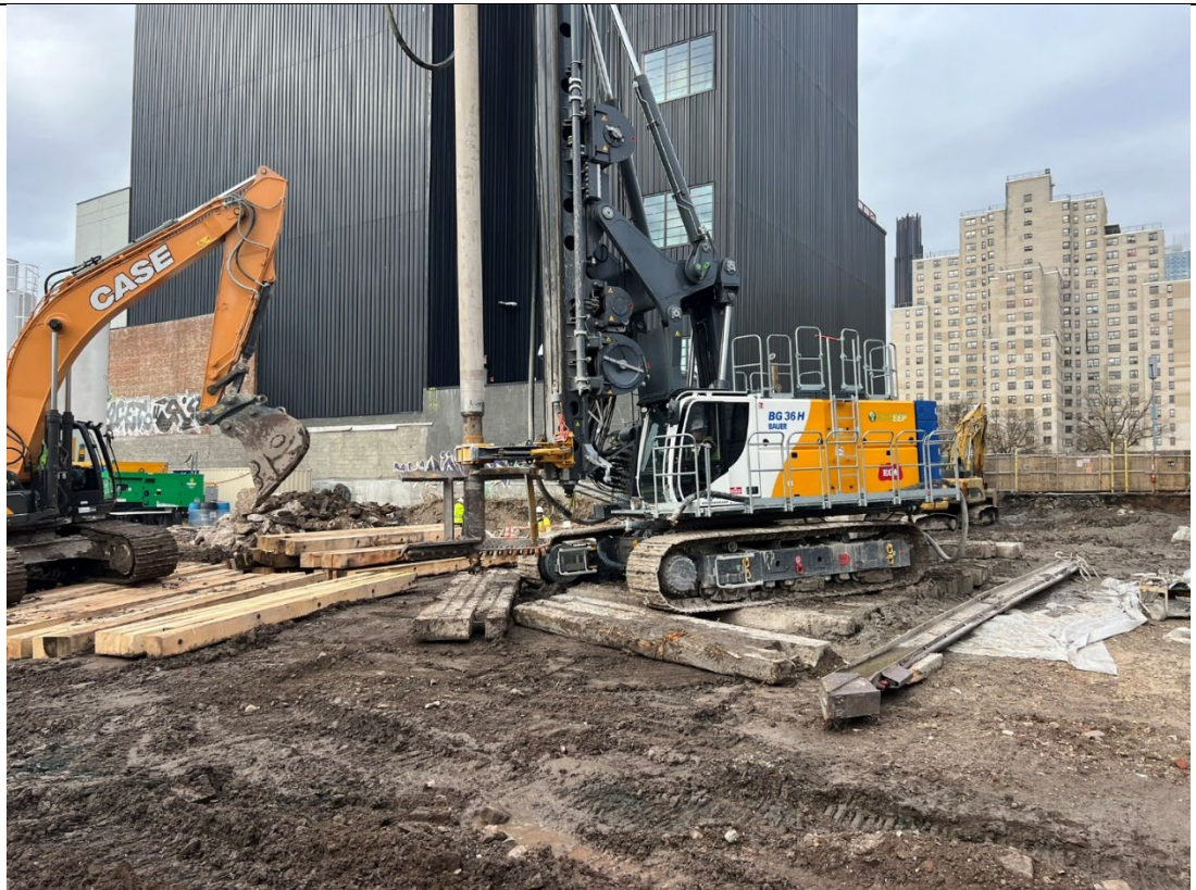
Photo 4- Representative photo of moving the drill rig.
