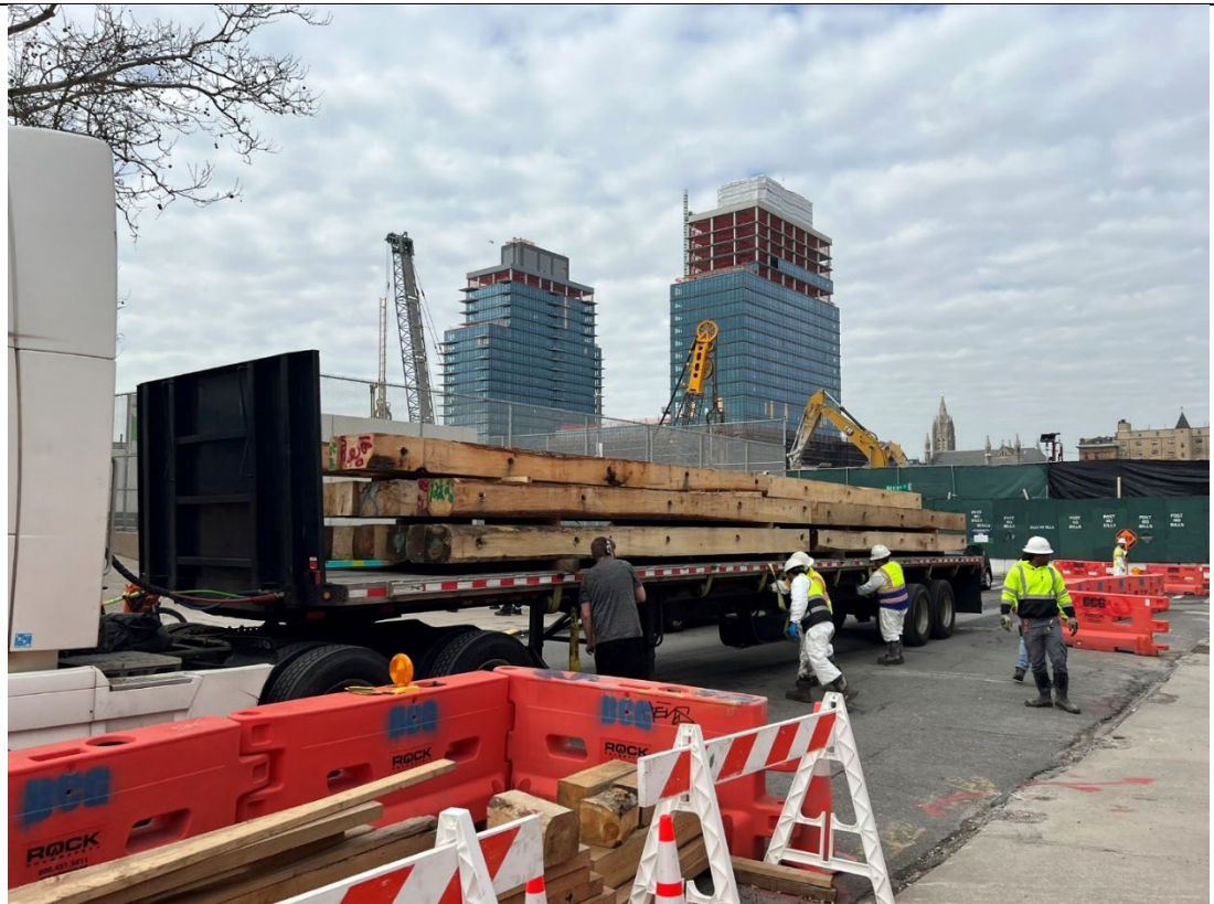
Photo 2 – Representative photo of additional drilling mats being delivered to the site.
