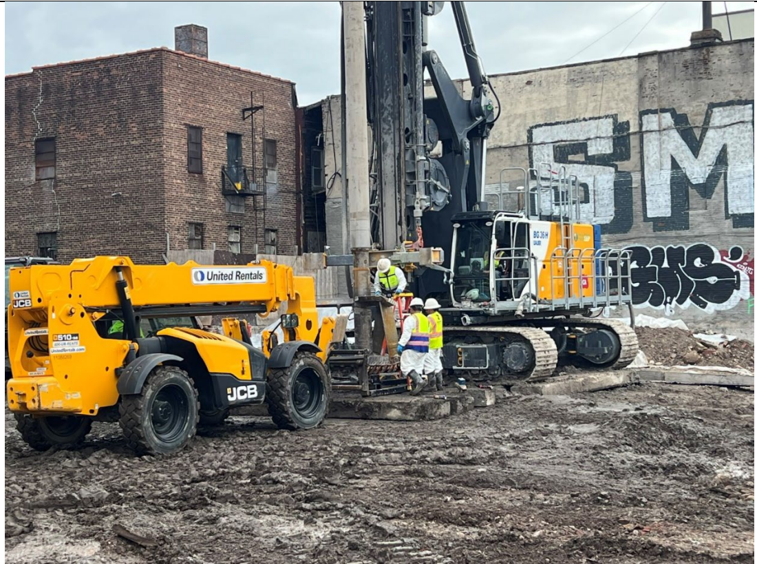
Photo 1- Representative photo of removing the 6' auger from the drill rig.
