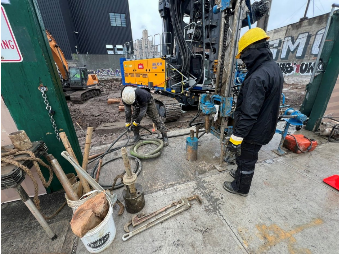
Photo 1- Representative photo of GES drilling a soil boring in the sidewalk.
