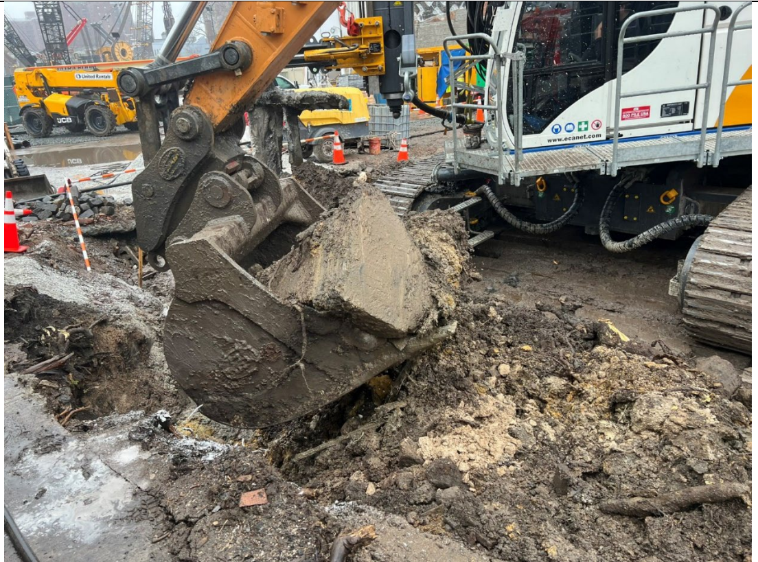
Photo 3- Representative photo of obstructions being removed from ISS column locations.
