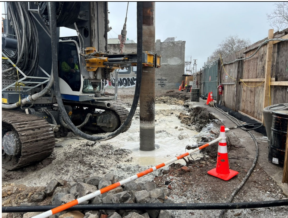
Photo 2- Representative photo of drilling an ISS .
