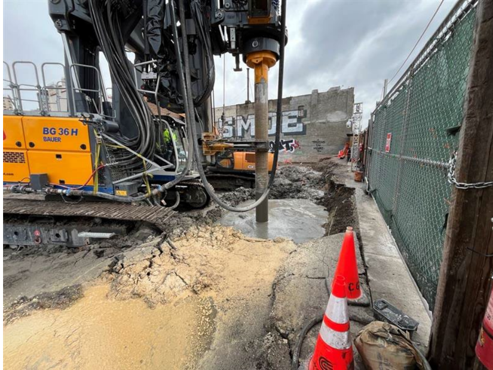
Photo 3- Additional representative photo of drilling ISS column.
