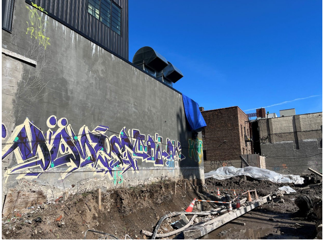
Photo 1- Representative photo of Cascade waterproofing the adjacent building.
