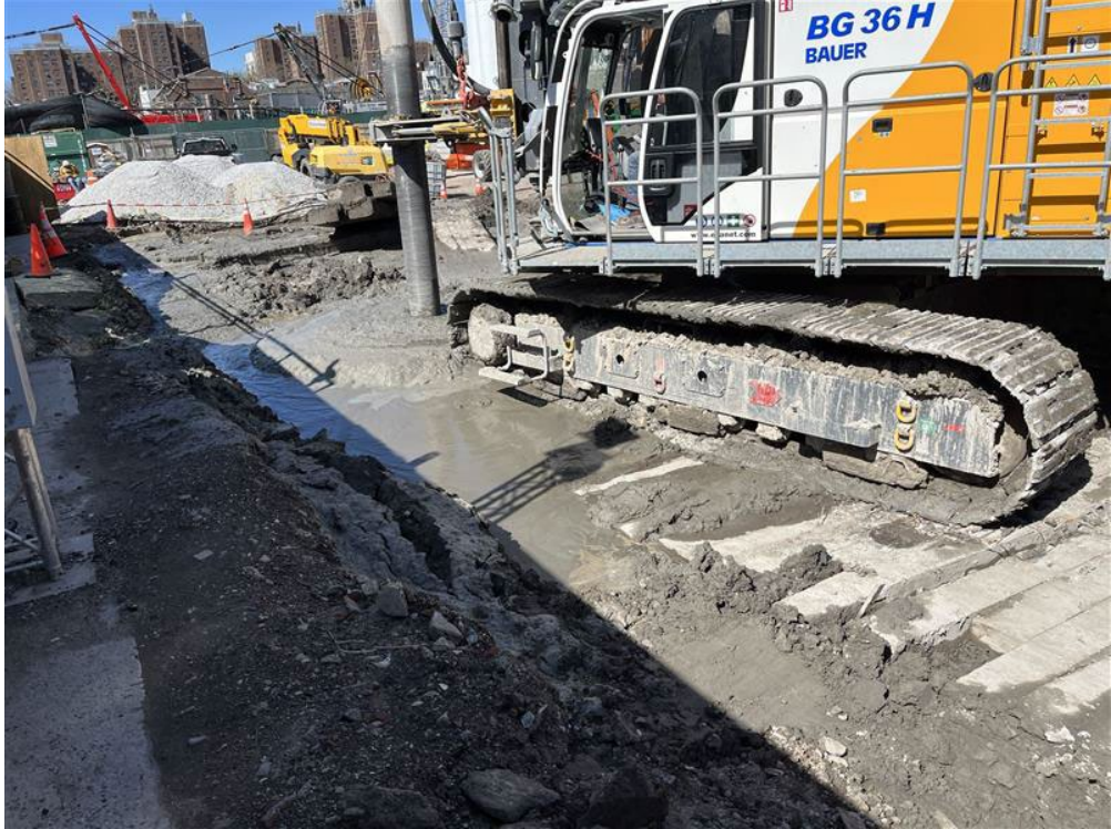
Photo 1- Representative photo of drilling ISS column.
