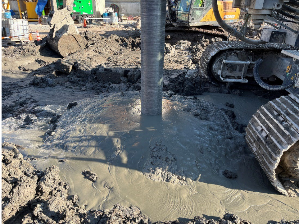
Photo 1- Representative photo of drilling ISS column.
