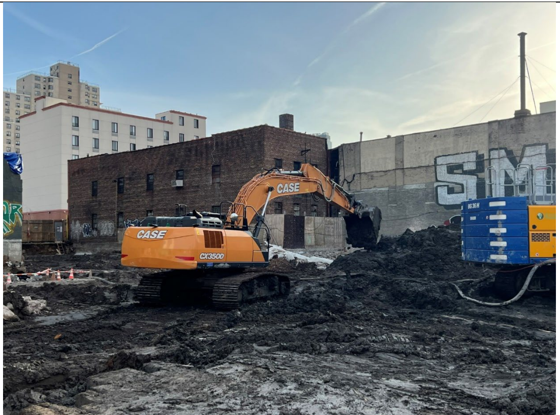
Photo 2- Representative photo of stockpiling swell material from ISS columns.
