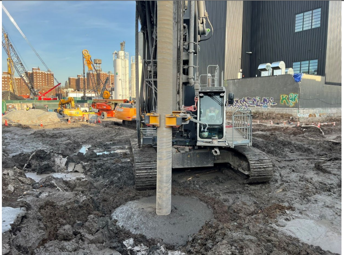
Photo 1- Representative photo of drilling ISS column.
