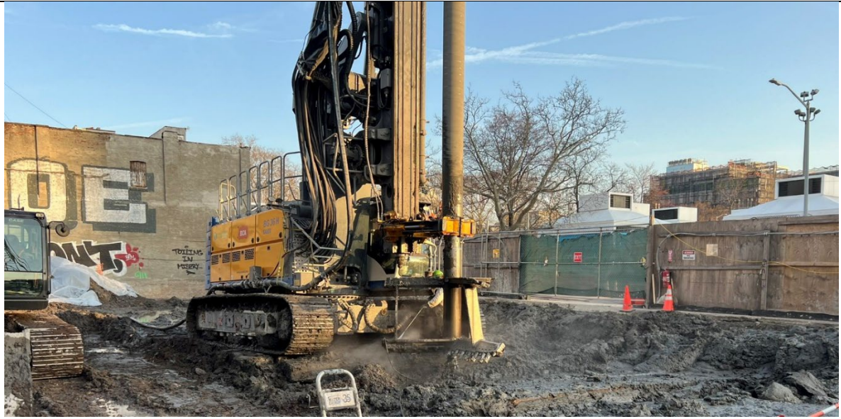
Photo 3- Representative photo of auger decontamination at the end of site activities.
