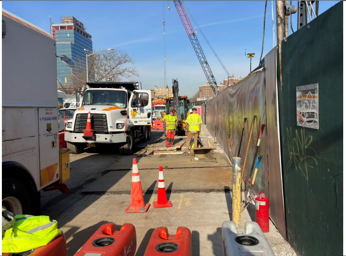
Photo 5- Representative photo of National Grid working in the sidewalk.
