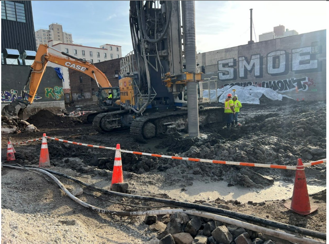
Photo 1- Representative photo of drilling ISS column.
