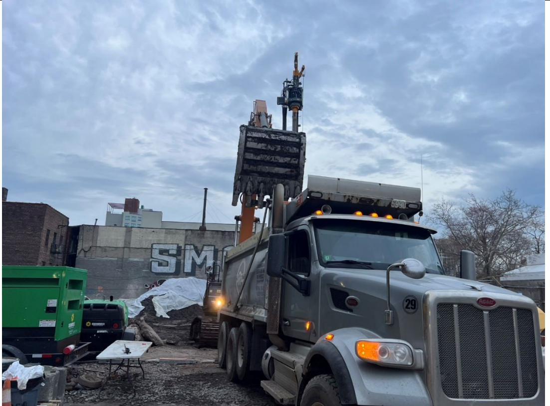
Photo 2- Representative photo of concrete being removed for offsite disposal.
