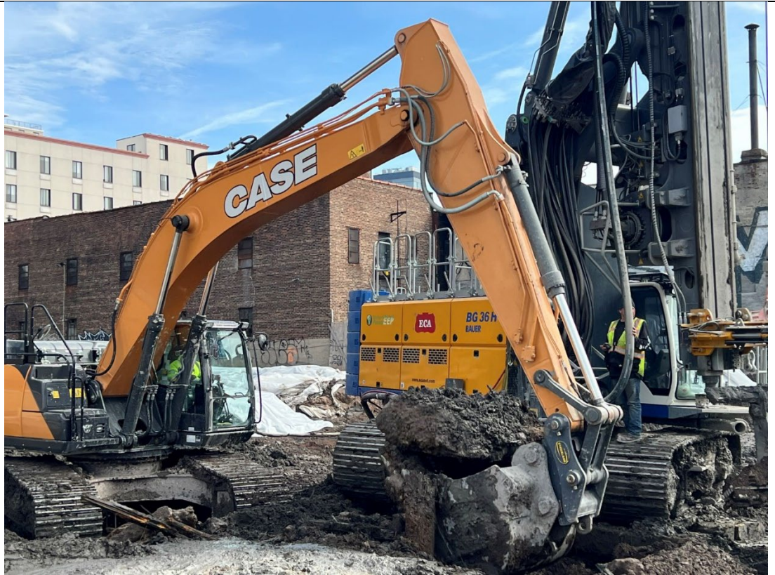
Photo 5- Representative photo of shallow obstruction being removed from ISS column.
