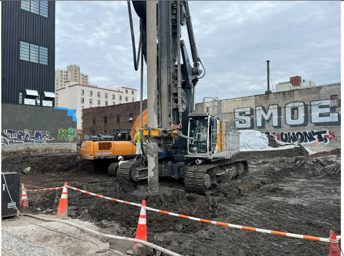
Photo 1- Representative photo of drilling ISS column.
