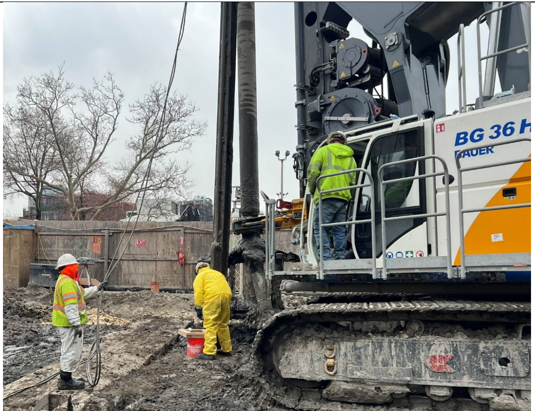
Photo 2- Representative photo collecting a wet mix sample.
