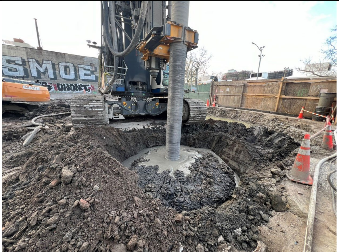
Photo 1- Representative photo of drilling ISS column.
