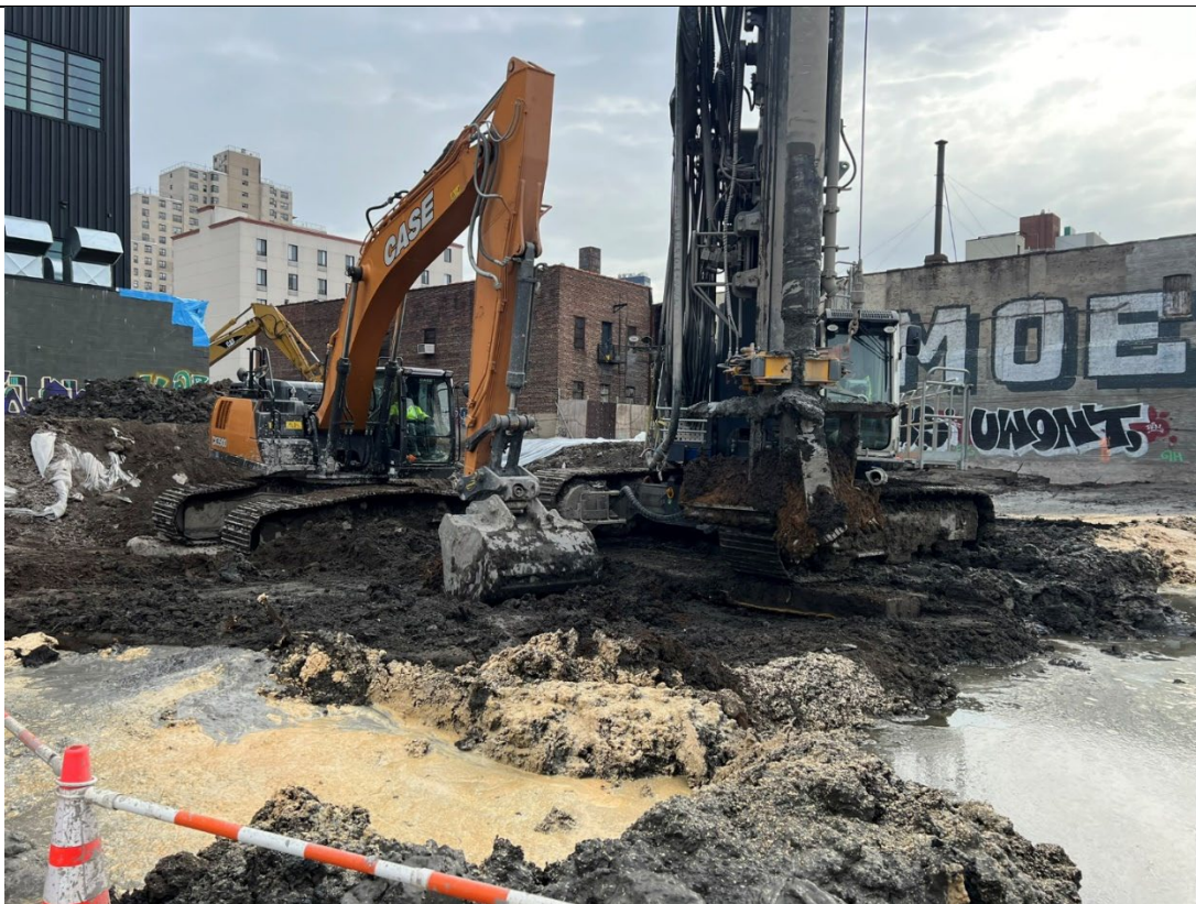
Photo 5- Representative photo of removing an obstruction from an ISS column.
