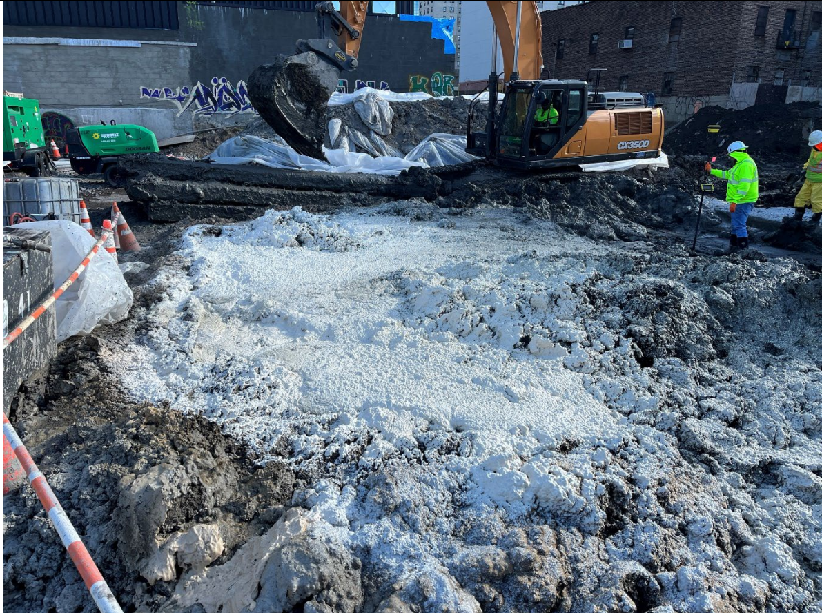
Photo 2- Representative photo of ATMOS foam sprayed over swell material.
