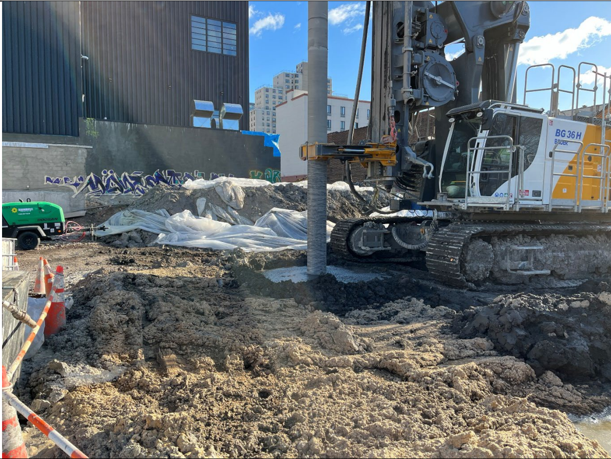
Photo 1- Representative photo of drilling ISS column.
