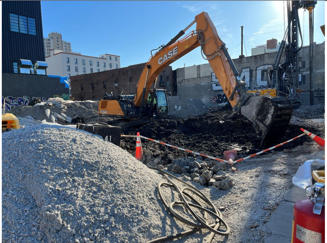
Photo 3- Representative photo of stockpiling swell material to prepare for core drilling.
