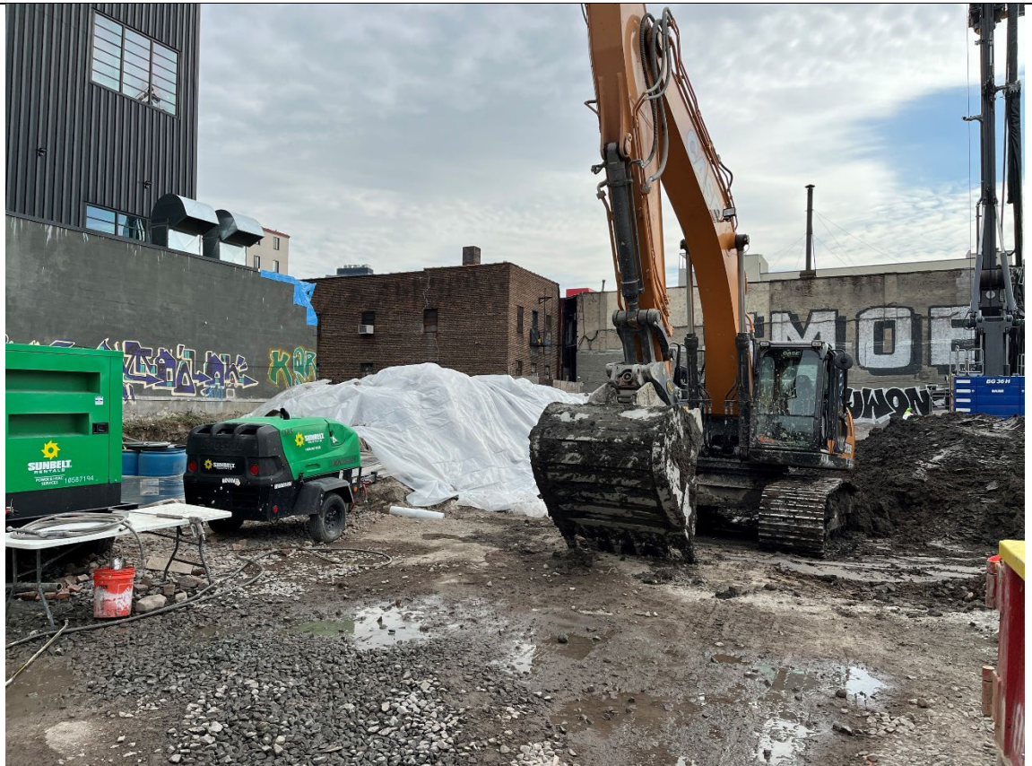
Photo 4- Representative photo of swell stockpile securely covered in poly sheeting.
