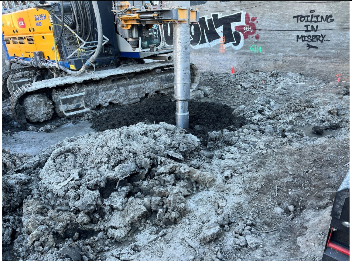
Photo 1- Representative photo of drilling ISS column.
