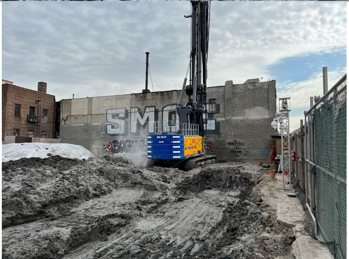
Photo 2- Representative photo of drill rig decontamination.
