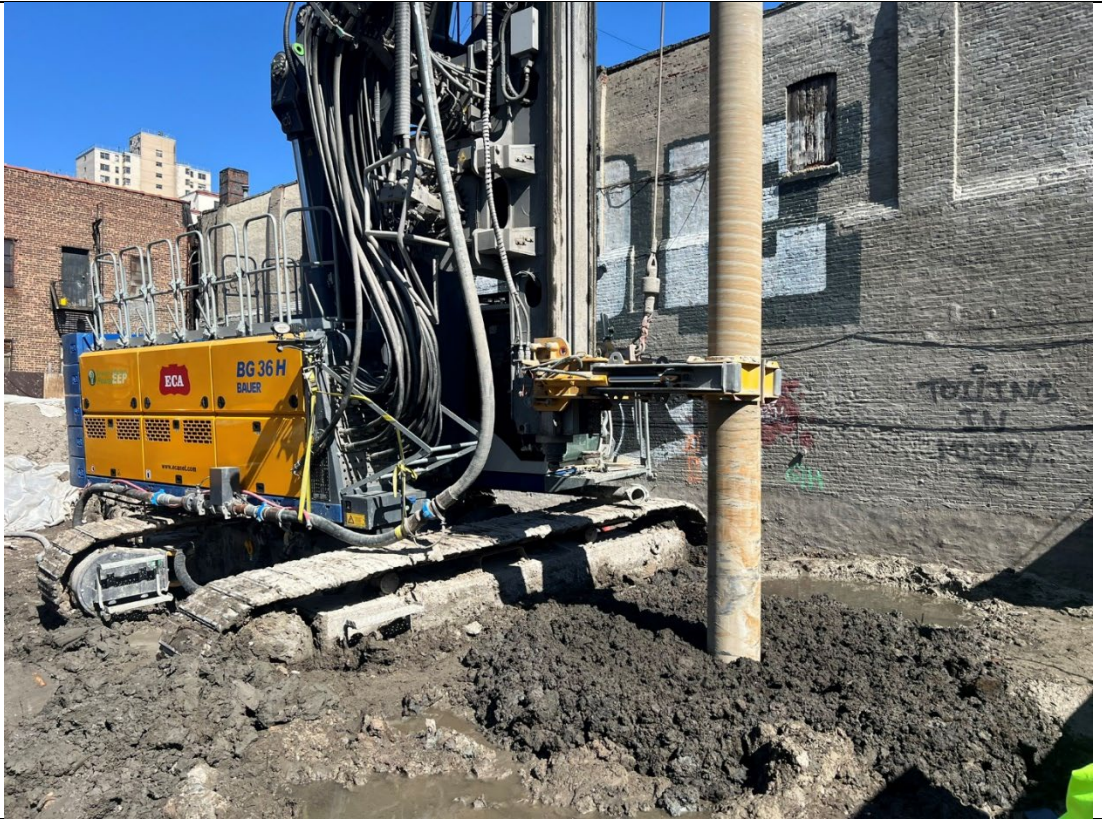
Photo 1- Representative photo of drilling ISS column.
