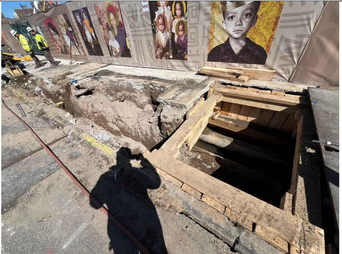
Photo 4- Representative photo of National Grid work in the sidewalk.
