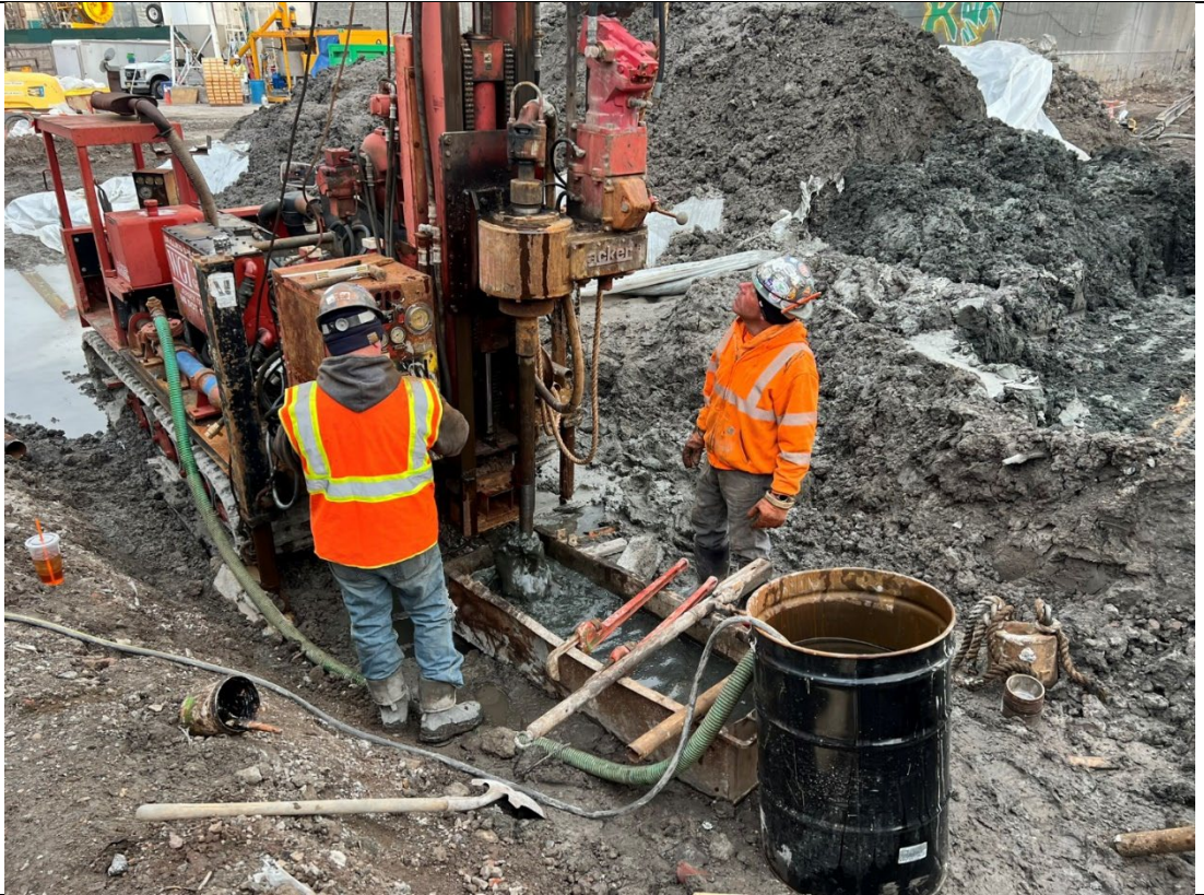
Photo 1- Representative photo of coring 24-25 OL.
