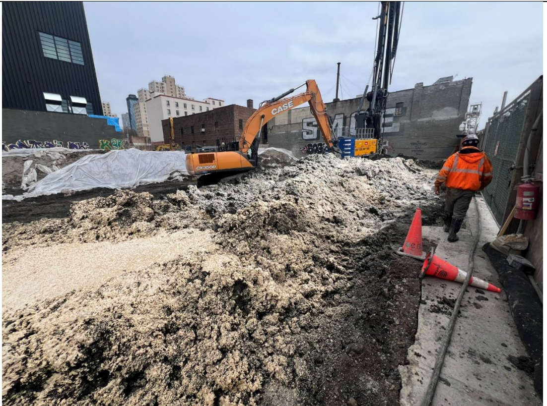
Photo 4- Representative photo of swell pile covered with ATMOS foam.
