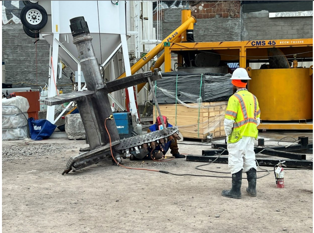
Photo 3- Representative photo of maintenance and repair on the 8' auger.
