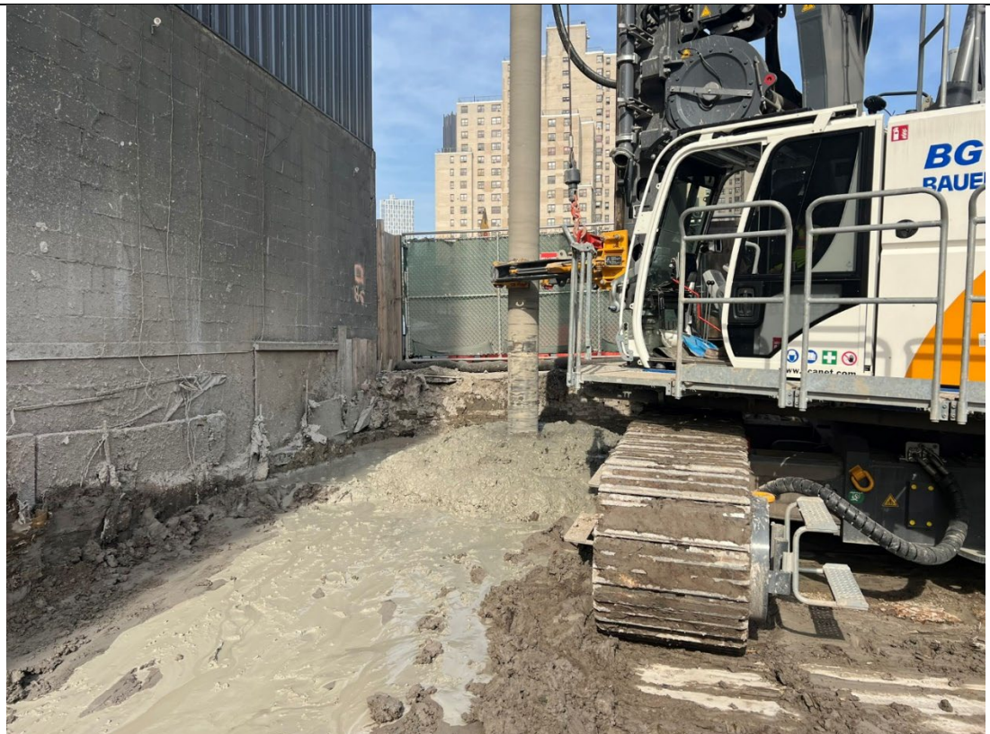
Photo 2 – Representative photo of ISS column installation.
