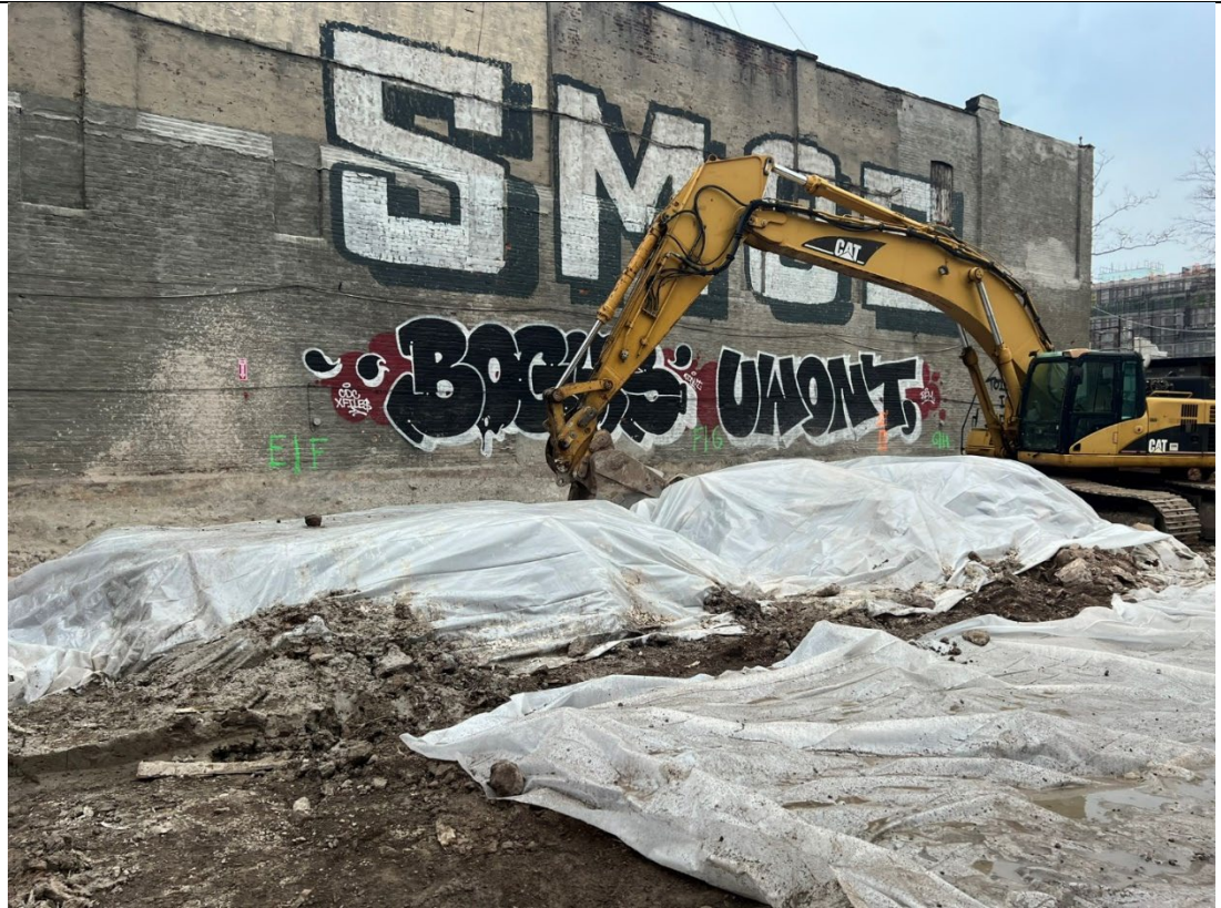
Photo 5- Representative photo of stockpile covered at the end of the work day.
